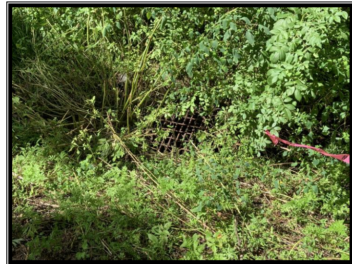
Photograph 16: Drop inlet located within Wetland A.
