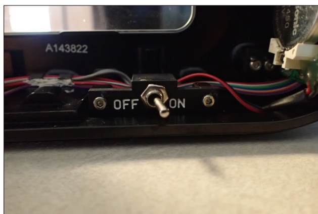
Figure 8. Moisture detector alarm switch in the ON position
