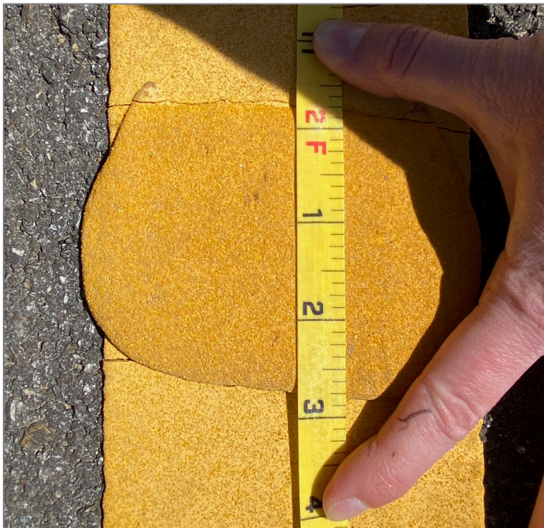
Figure 24. NATR RPS installation example 2. NPS / KELSEY WHITE
