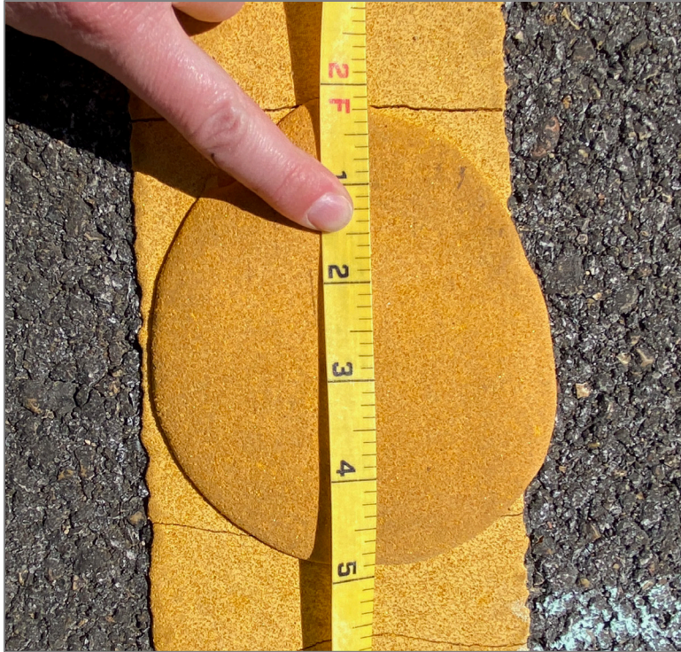
Figure 23. NATR RPS installation example 1. NPS / KELSEY WHITE
