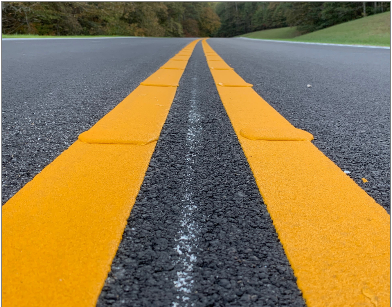
Photograph of roadway center line raised profile striping. NPS / KELSEY WHITE
