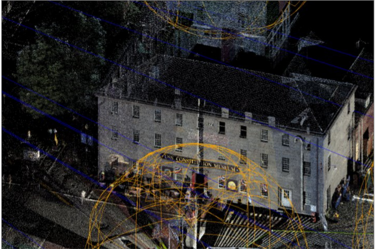
Figure 6. Point cloud view of the USS Constitution Museum at Charlestown Navy Yard, Boston National Historical Park. The image is entirely generated by points and colorized by the panoramic photographs taken before the scan. The orange sphere represents the path of the scanner while scanning.
