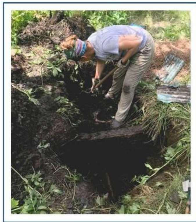
Figure 5. Pipe shown exiting spring box on north side; EL is in interior of box, re-excavating it on July 26.
