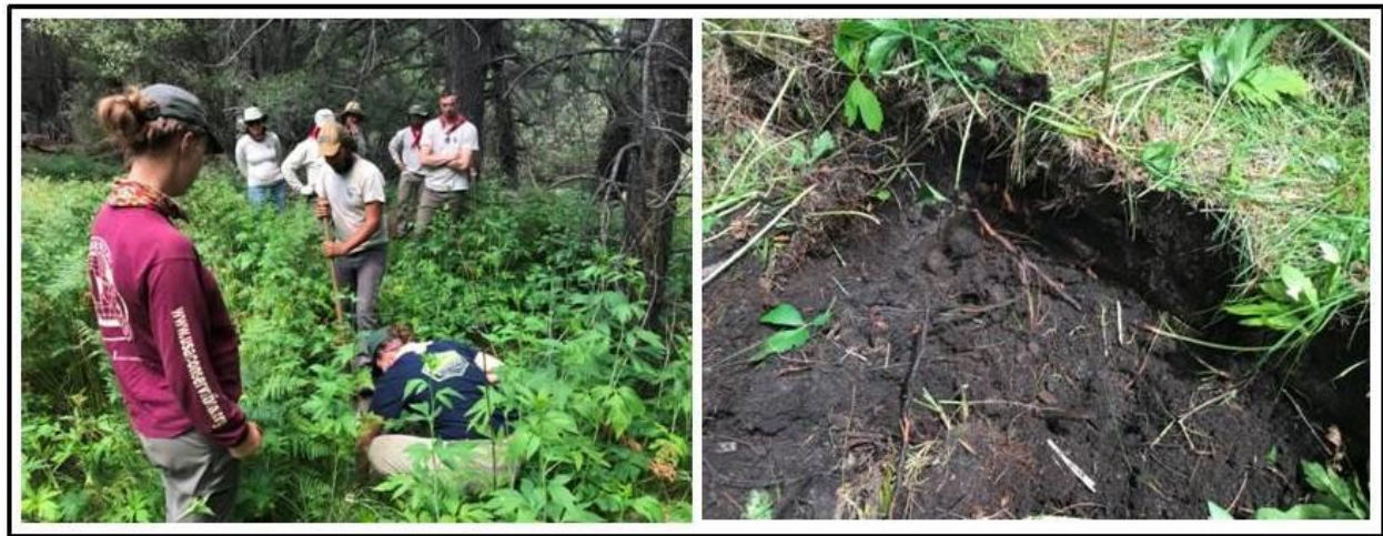
Figure 3. Initial excavation of spring box, June 24, showing some of the materials removed from the box that were apparently used to fill it when the spring was buried in the 1980s.
