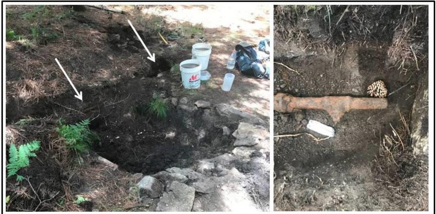
Figure 6. Left: arrows indicate location of pipe running just uphill of current Spud Rock Spring, approximately 20 m north of spring box. Right: pipe where it has been cut and lies at base of foundation of former water tank, also indicated by right-hand arrow in left figure.
