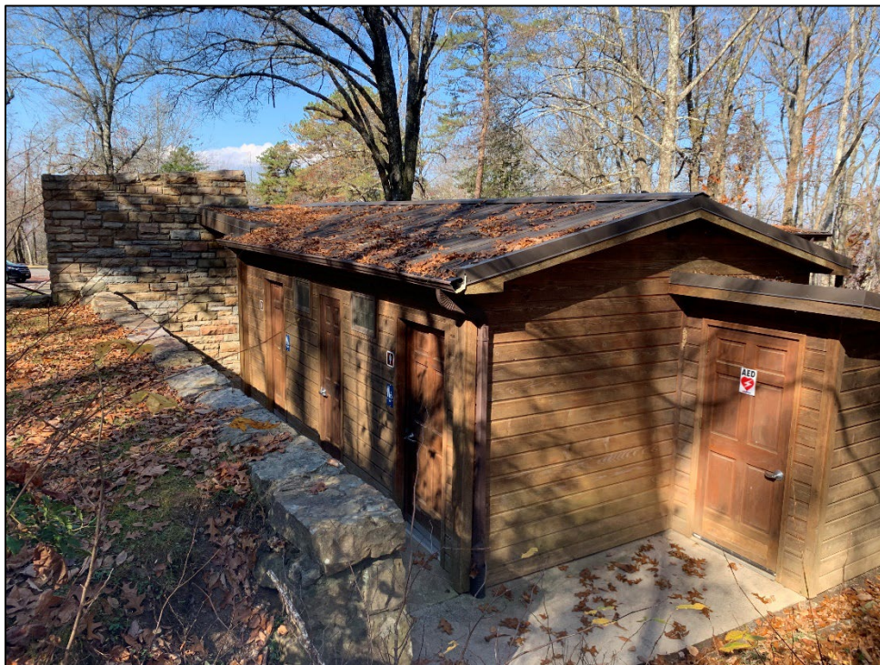
Photograph 11. View of the wood frame restrooms on the rear of the Information Shelter and Comfort Station building, facing west.
