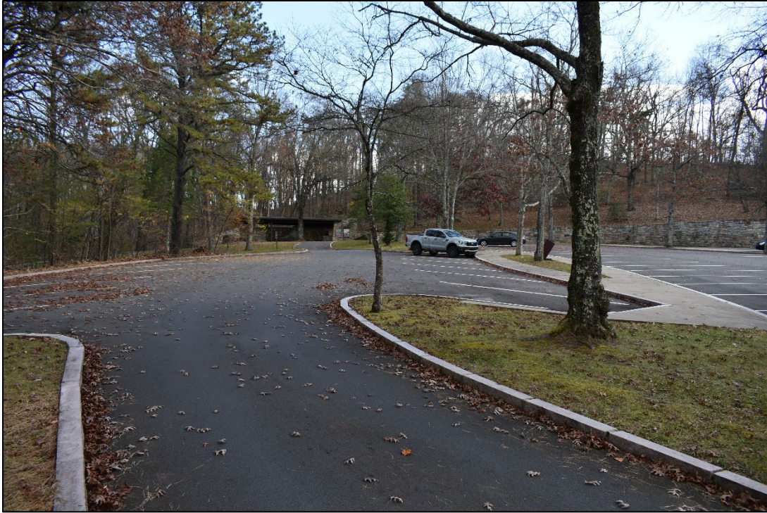
Photograph 12. Overview of the Pinnacle Parking Area, facing east.
