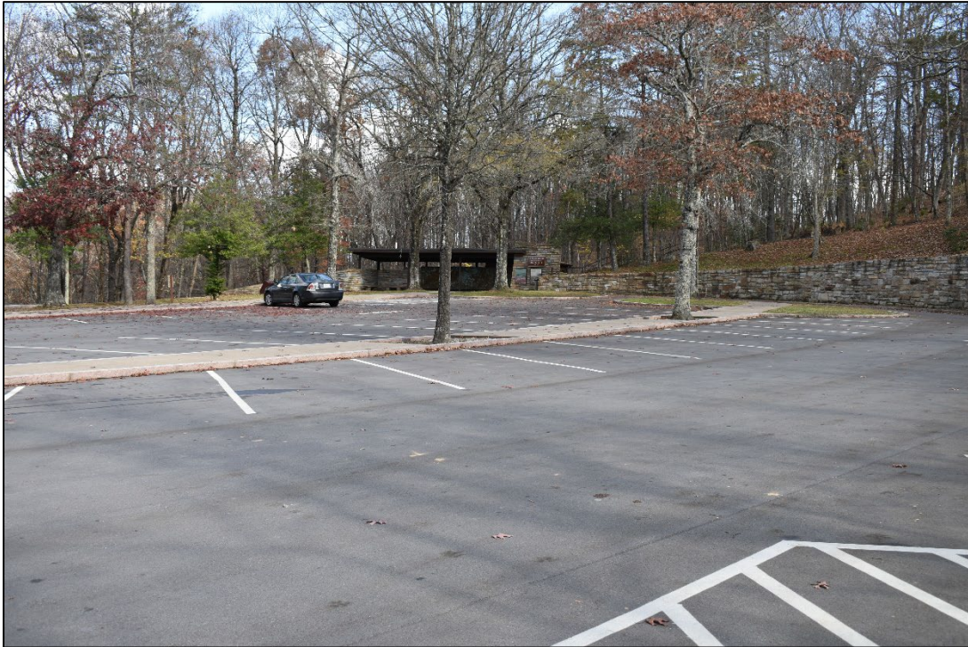
Photograph 4. Overview of the Pinnacle Parking Area, showing its relationship to the Interpretive Shelter and Comfort Station, facing east.
