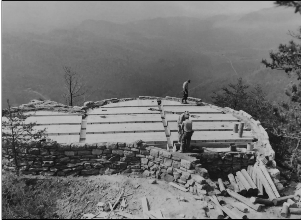
Figure 10. Construction of the Pinnacle Overlook Terrace, taken in April 1956 (Photograph on file at the Cumberland Gap National Historical Park archives, Middlesboro, Kentucky [Classification No. 978, Negative No. 2461]).
