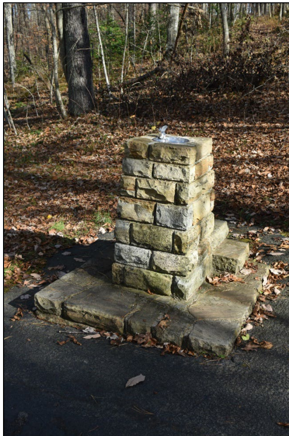
Photograph 16. Current view of the drinking fountain, facing north.
