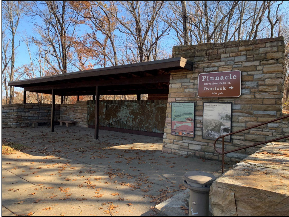
Photograph 9. View of the Interpretive Shelter and Comfort Station, facing southeast.
