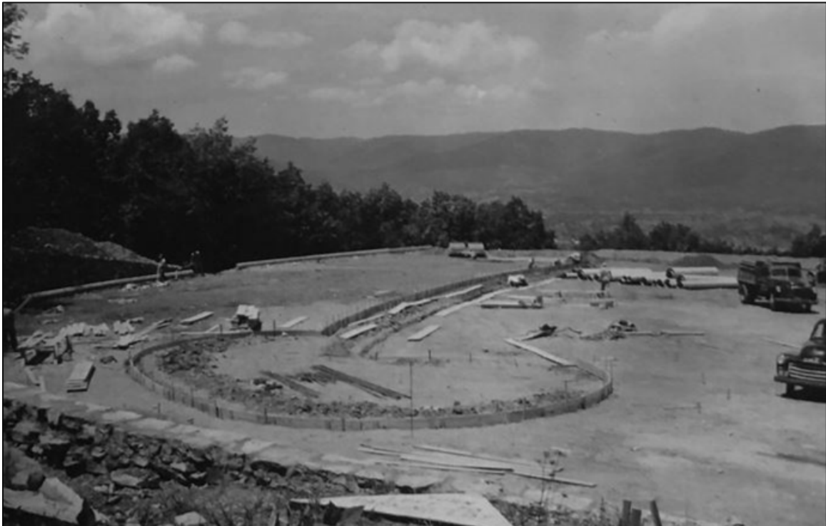
Figure 9. Pinnacle Parking Area under construction, ca. 1956 (Image reprinted from National Park Service 1956).
