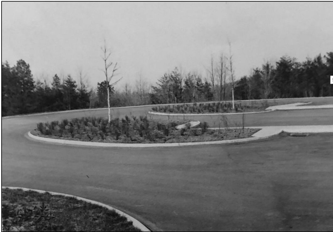
Figure 13. Landscaping in the Pinnacle Parking Area, shortly after completion, ca. 1958 (Image reprinted from National Park Service 1958b).
