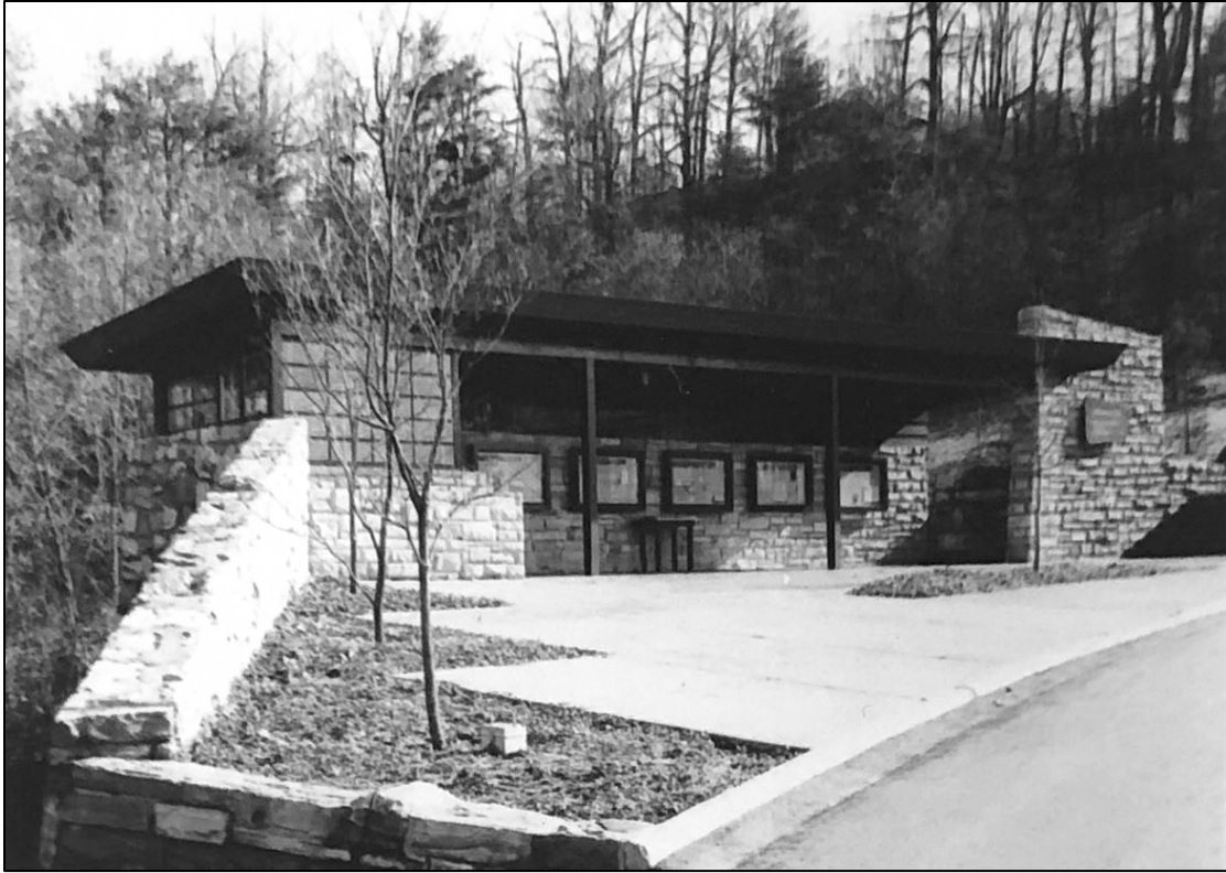
Figure 16. Photograph of the Interpretive Shelter and Comfort Station shortly after its completion, ca. 1958 (Image reprinted from National Park Service 1958).
