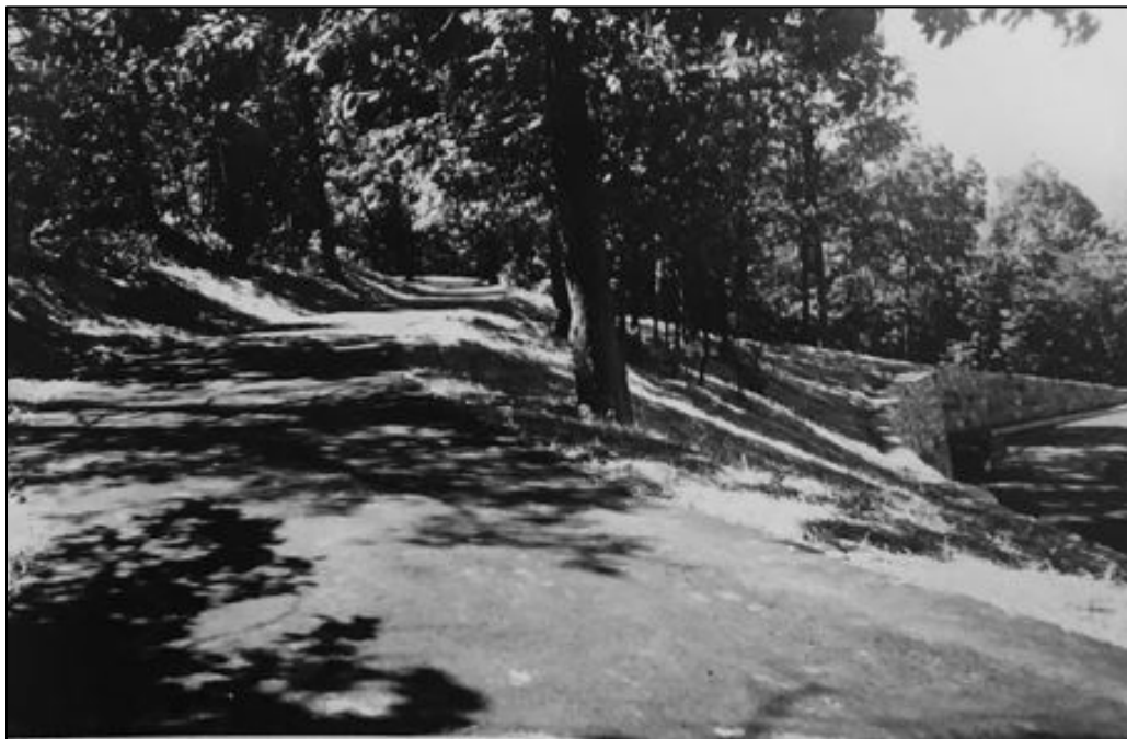
Figure 23. Pinnacle Loop Trail shortly after its completion, ca. 1956 (Image reprinted from National Park Service 1956).
