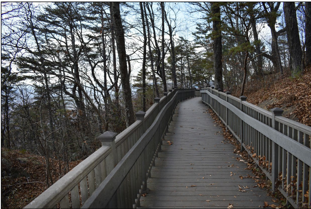
Photograph 7. View of composite boardwalk and railing along the handicap accessible portion of the Pinnacle Loop Trail, facing northeast.
