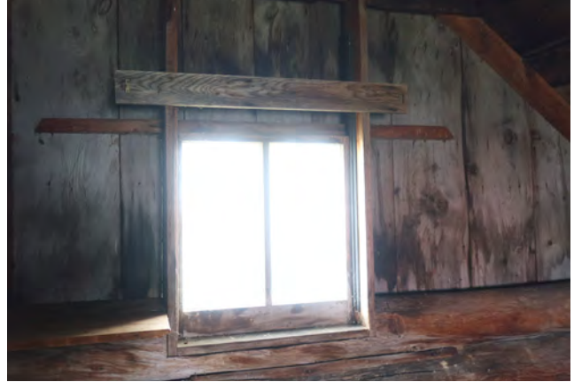
Figure 4-18. Second floor north window, interior (source: Anderson Hallas, 2024).
