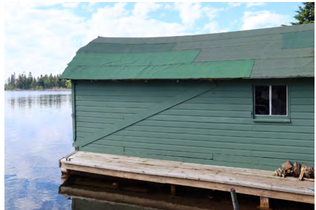
Figure 3-11. Tongue and groove 1x12 board on east façade (source: Anderson Hallas, 2024).
