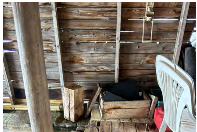
Figure 3-12. Interior face of west wall (source: Anderson Hallas, 2024).
