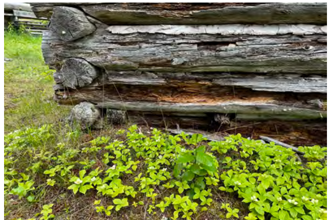
Figure 4-31. First-floor beam ends exposed to exterior and in close proximity to soil (source: JVA, 2024).
