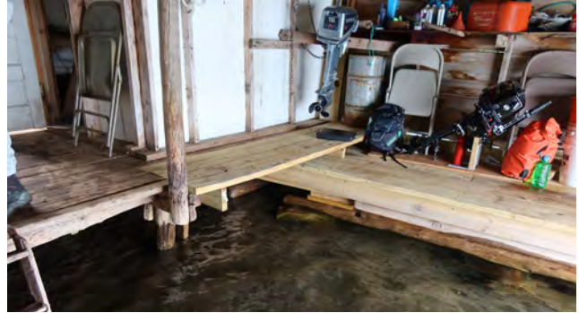
Figure 3-23. Exposed floor decking; looking northwest from southeast corner (source: Anderson Hallas, 2024).
