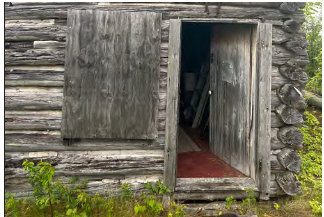
Figure 4-21. Entry door and boarded window at south façade (source: Anderson Hallas, 2024).
