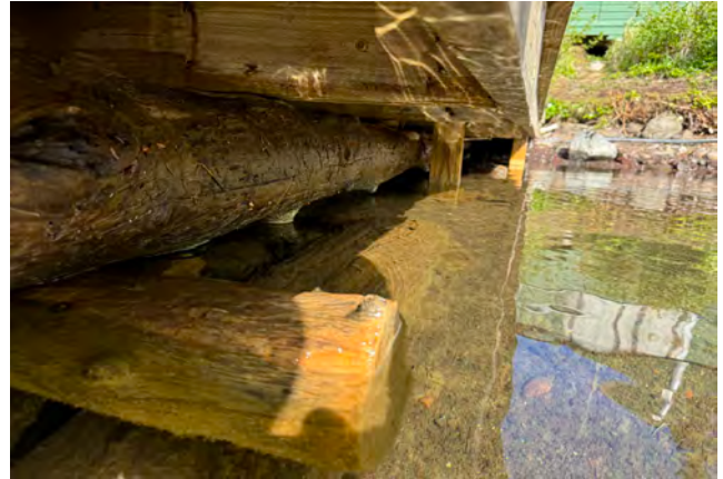
Figure 3-29. Dimensional-lumber floor framing on log cribs (source: JVA, 2024).
