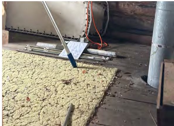
Figure 4-27. Second floor decking and carpet (source: Anderson Hallas, 2024).
