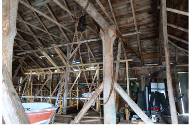
Figure 2-25. East end of boat hoist (source: Anderson Hallas, 2024).
