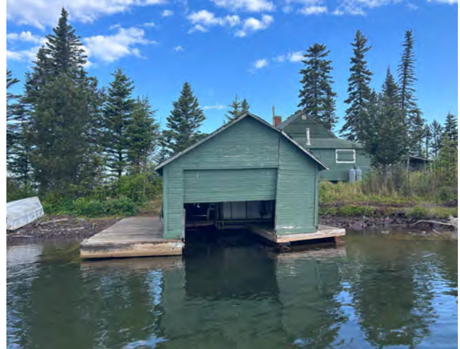
Figure 1-8. Small Barnum Boat House (source: Anderson Hallas, 2024).
