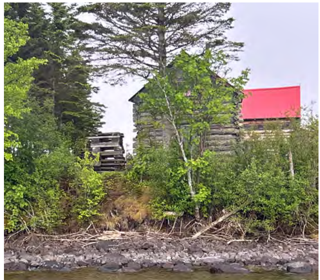
Figure 4-10. Shoreline vegetation provides cliff stabilization while obstructing views from inside Johns Log Cabin to Washington Harbor and Thompson Island (source: Anderson Hallas, 2024).
