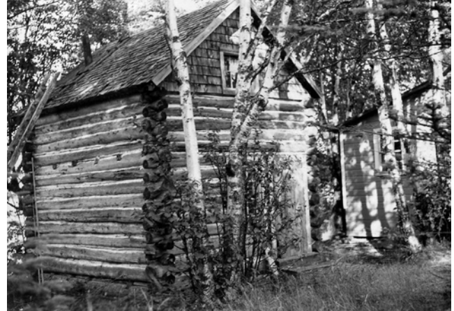
Figure 4-15. Barnum Log House, c. 1935 (source: ISRO Archives).
