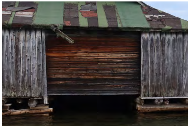
Figure 2-20. Boat door on west façade (source: Anderson Hallas, 2024).
