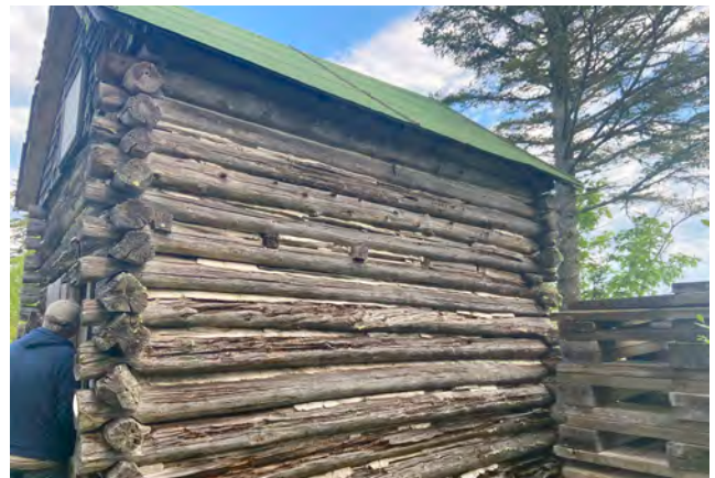
Figure 4-12. Log construction viewed at east façade (source: Anderson Hallas, 2024).
