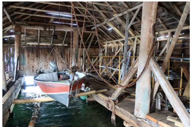
Figure 2-11. Interior of Boat House, facing west (source: Anderson Hallas, 2024).
