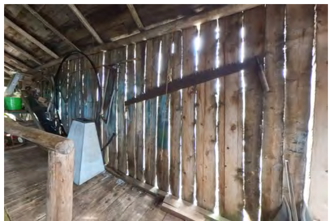
Figure 2-35. East wall framing (source: JVA, 2024).
