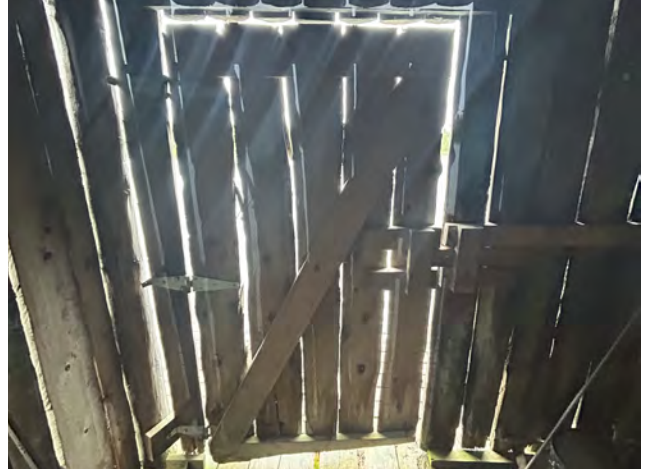
Figure 2-19. South door interior (source: Anderson Hallas, 2024).
