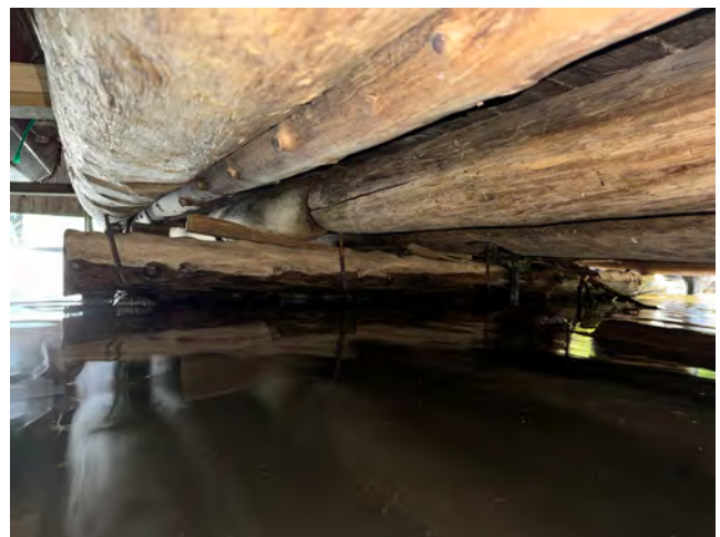
Figure 2-30. Log floor framing supported on cribs (source: JVA, 2024).
