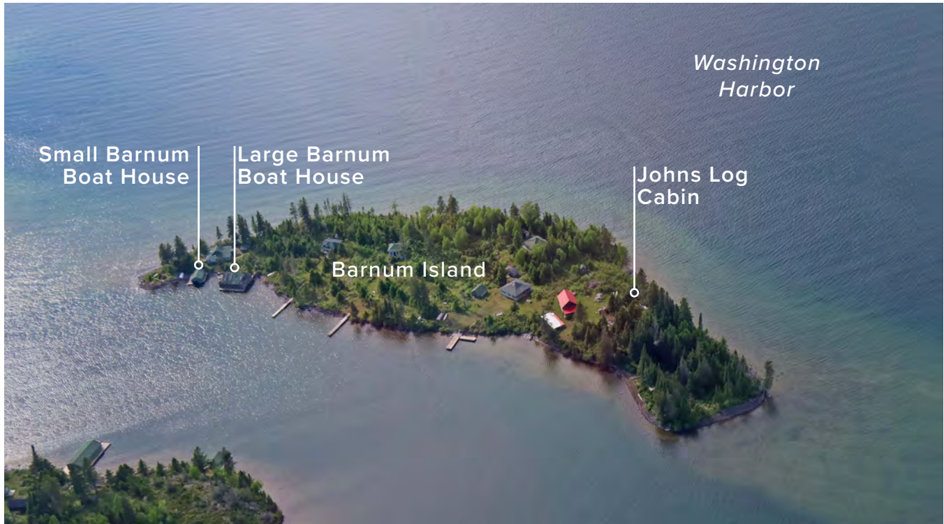
Figure 1-2. The study area includes Small Barnum Boat House, Large Barnum Boat House, Johns Log Cabin, and the cultural landscape associated with each building (source: Anderson Hallas, 2024).
