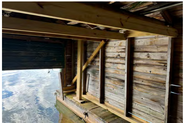
Figure 3-32. Recently installed 2x6 ties at the top of the wall framing to stabilize the roof structure (source: JVA, 2024).
