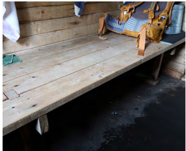
Figure 3-24. Sauna room flooring (source: Anderson Hallas, 2024).
