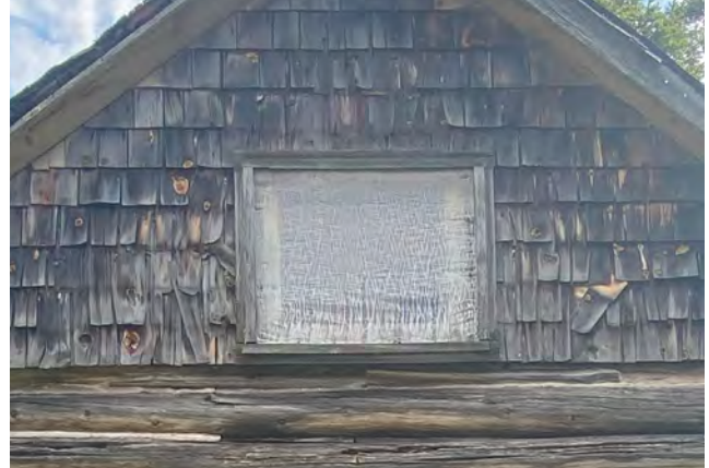
Figure 4-19. Second floor south window, exterior (source: Anderson Hallas, 2024).
