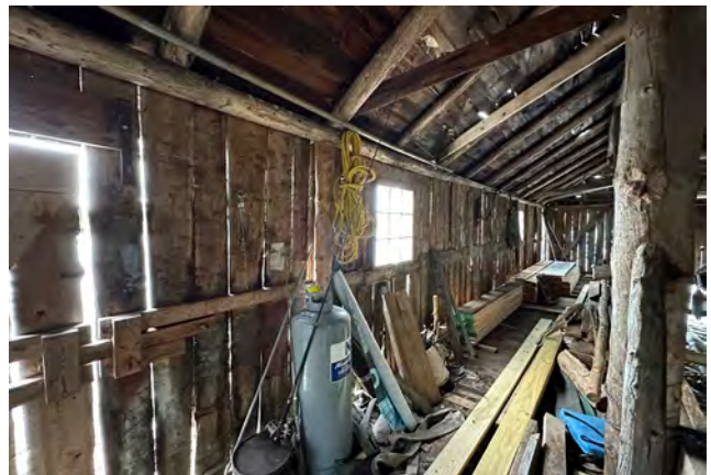
Figure 2-34. South wall framing (source: JVA, 2024).
