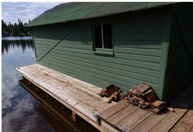
Figure 3-9. Wood deck along the east façade (source: Anderson Hallas, 2024).
