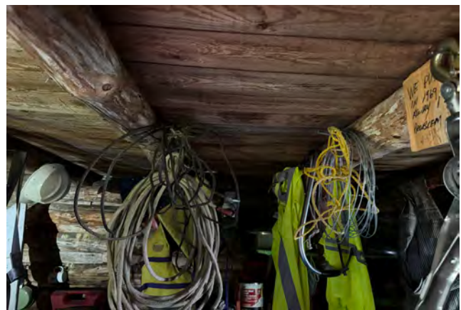
Figure 4-33. Second-floor beams (source: JVA, 2024).
