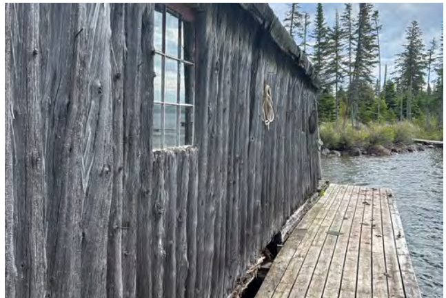
Figure 2-10. Vertical log slab cladding, south façade (source: Anderson Hallas, 2024).
