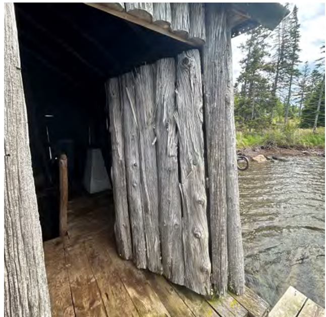
Figure 2-18. South door (source: Anderson Hallas, 2024).
