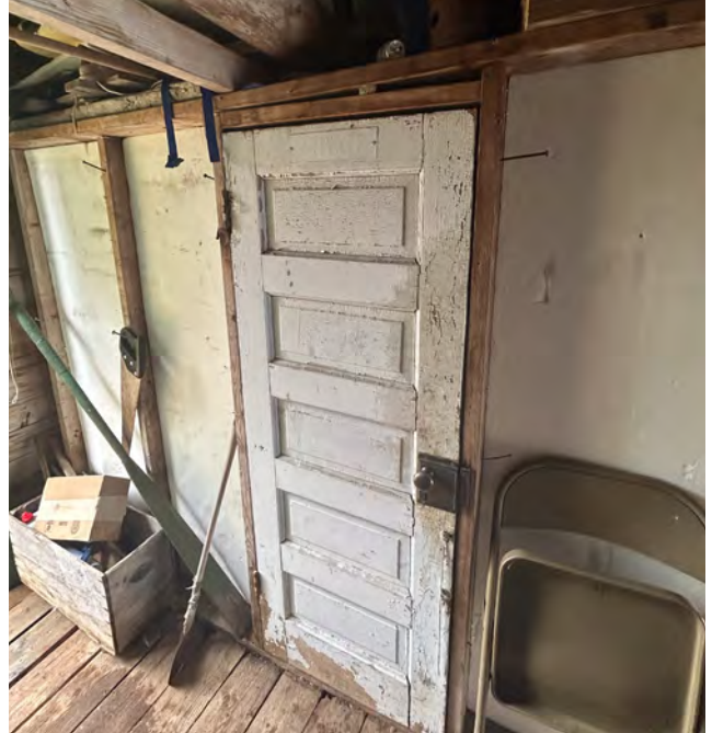
Figure 3-20. Interior door (source: Anderson Hallas, 2024).
