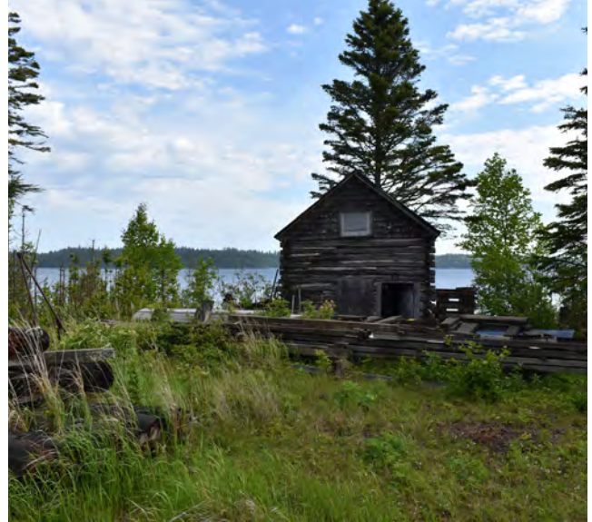
Figure 4-4. The historic setting is modified by the encroachment of vegetation into the clearing surrounding Johns Log Cabin and storage of building material (source: Mundus Bishop, 2024).
