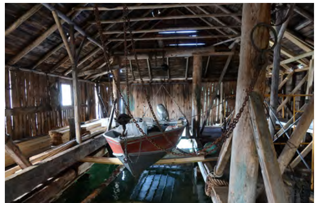
Figure 2-24. Large Barnum Boat House interior (source: Anderson Hallas, 2024).
