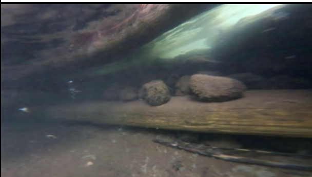
Figure 4. Loss of rock ballast (source: AMI, 2024).
