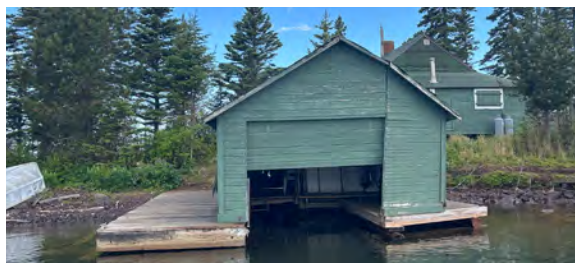
Figure 3-15. Boat door, exterior (source: Anderson Hallas, 2024).
