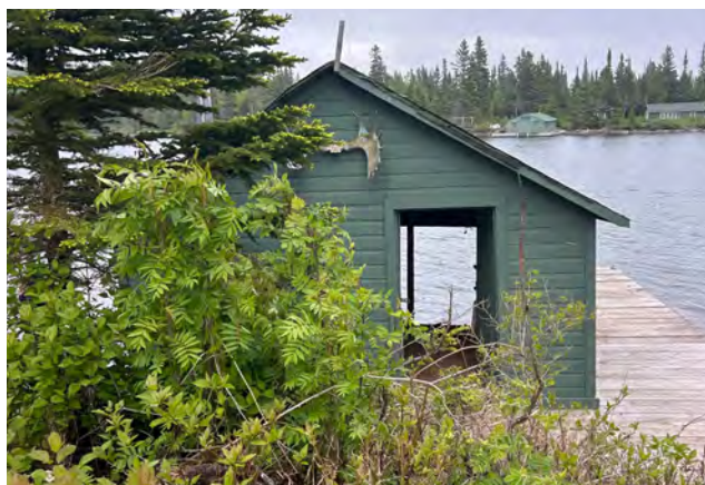
Figure 3-8. North façade (source: Anderson Hallas, 2024).
