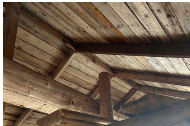
Figure 3-25. Exposed underside of roof structure (source: Anderson Hallas, 2024).
