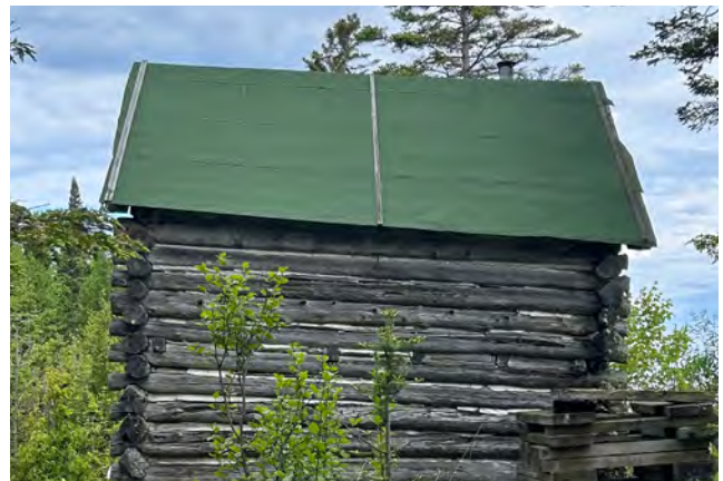
Figure 4-13. East slope of roof (source: Anderson Hallas, 2024).
