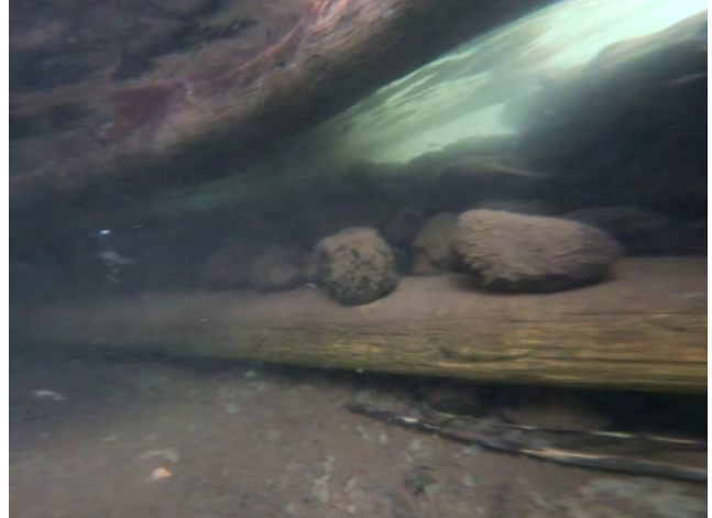
Figure 3-28. Loss of rock ballast (source: AMI, 2024).
