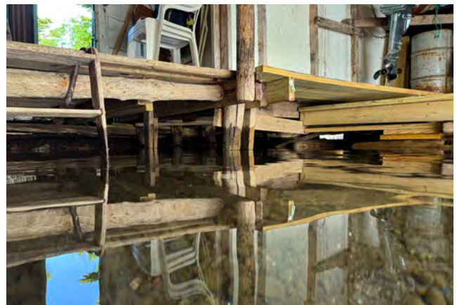
Figure 3-30. Floor framing at the north supported on cribs and posts (source: JVA, 2024).
