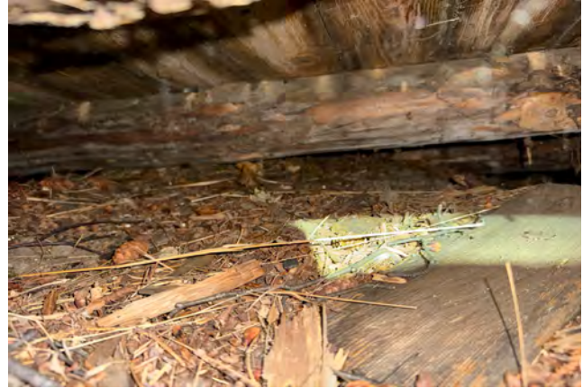
Figure 4-32. View of first-floor framing from a gap in the exterior logs (source: JVA, 2024).
