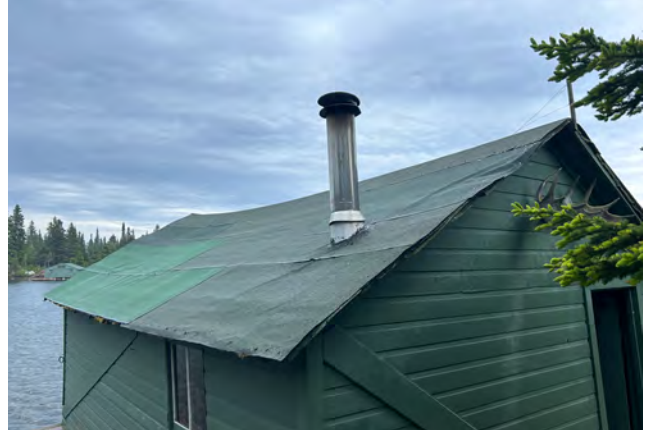
Figure 3-17. Roof viewed from northeast (source: Anderson Hallas, 2024).
