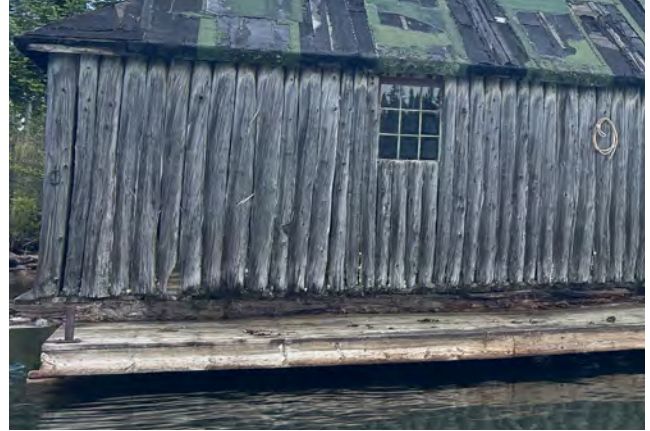
Figure 2-13. South exterior wall (source: Anderson Hallas, 2024).
