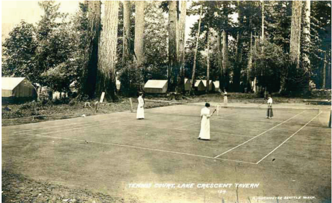
Figure 1: Lake Crescent Lodge tennis in the recreational lawn. Today, the absorption beds run north-south under the recreational lawn. A poured concrete tennis court is extant and contributes to the cultural landscape. (Clallam County Historical Society, 999.118.3)
