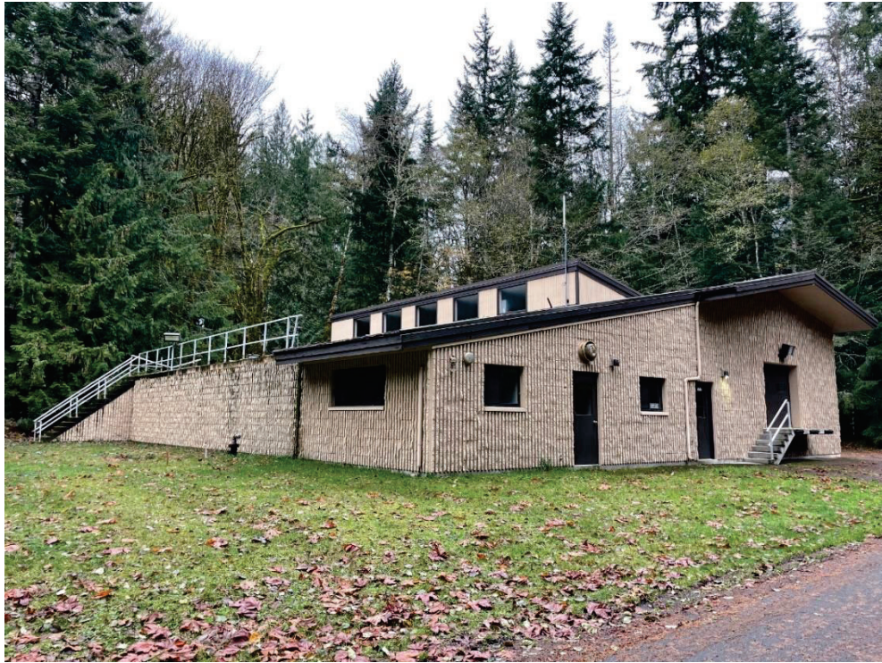
Photograph 1: East and South walls of Barnes Point Wastewater Treatment Plant (NPS/2024).
