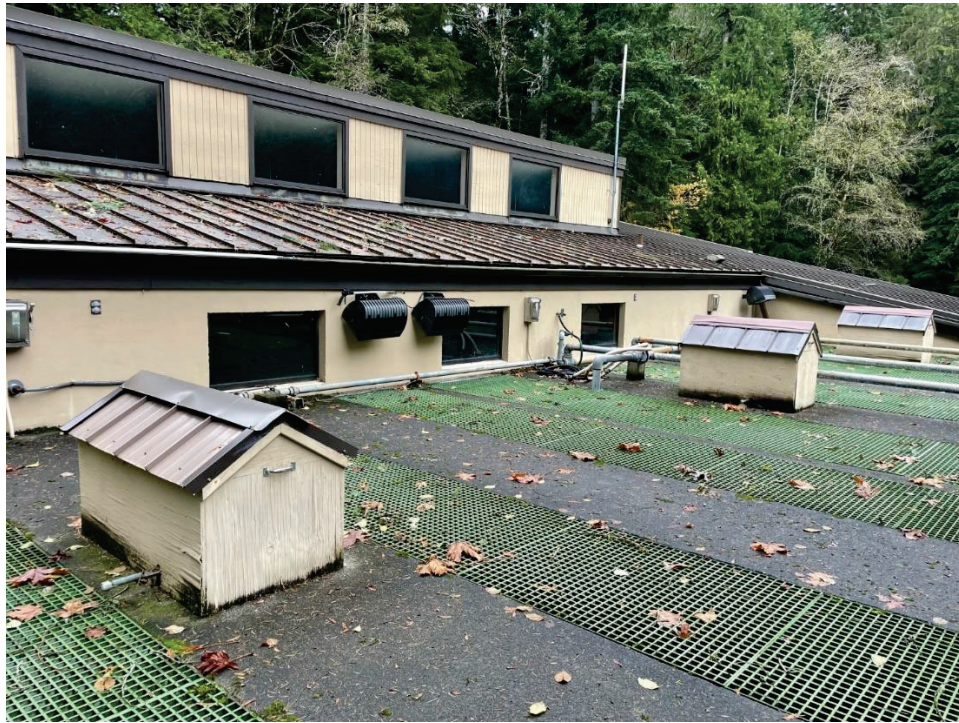
Photograph 3: Flat roof over tanks and clerestory windows of Barnes Point Wastewater Treatment Plant, looking northeast (NPS/2024).
