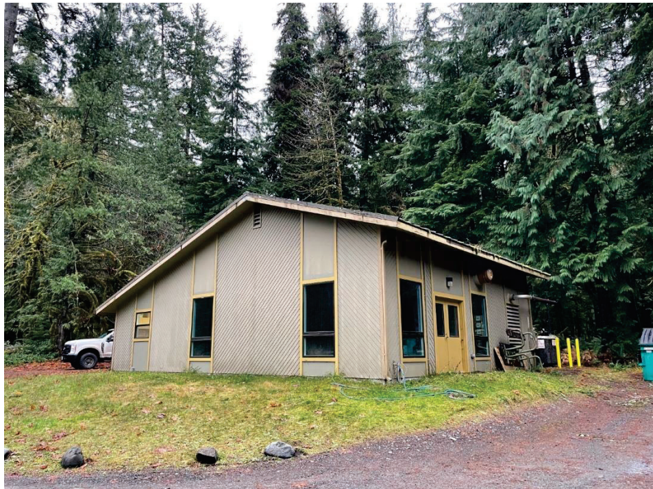
Photograph 8: North and West walls of the Barnes Point Water Treatment Plant at Rosemary Inn Campus, looking south (NPS/2024).
