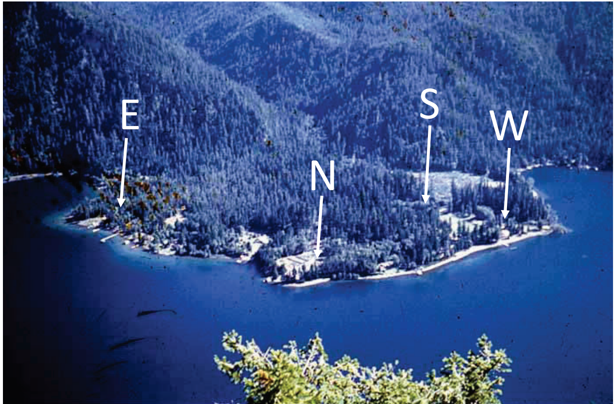
Figure 11: Barnes Point, looking south, with water and wastewater treatment key points located. (NPS 1991)
