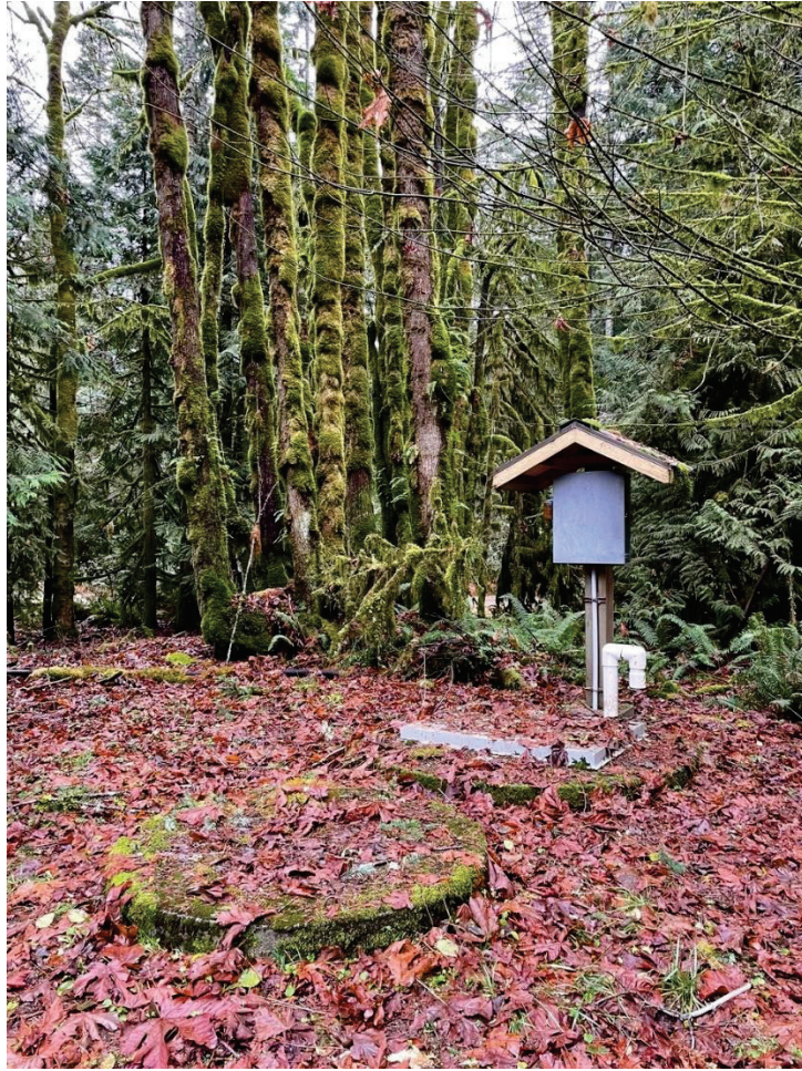
Photograph 5: Lift Station and valve vault west of Wastewater Treatment Plant, looking west (NPS/2024).
