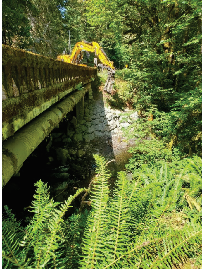
Photograph 6: Insulated pipe running along the west bridge beam as it crosses Barnes Creek, looking south (NPS/2020).
