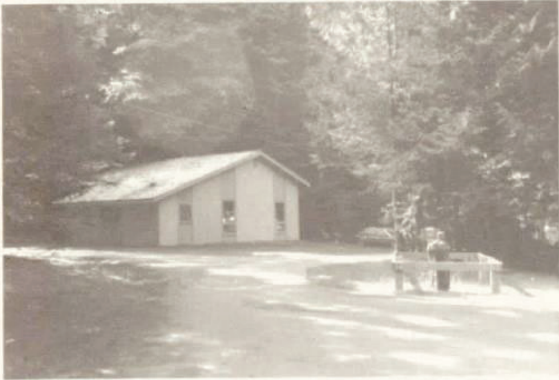
Fig. 40 Water treatment plant and one of two wells outside the gate. Drew Rocker, National Park Service, 1985.
