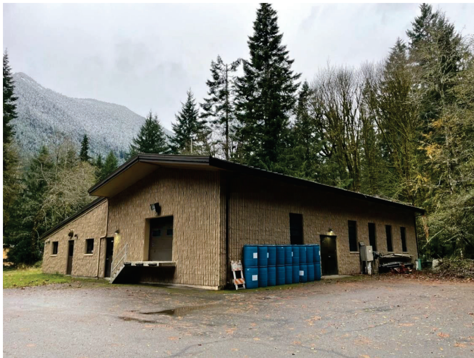
Photograph 2: East and North walls of Barnes Point Wastewater Treatment Plant (NPS/2024).
