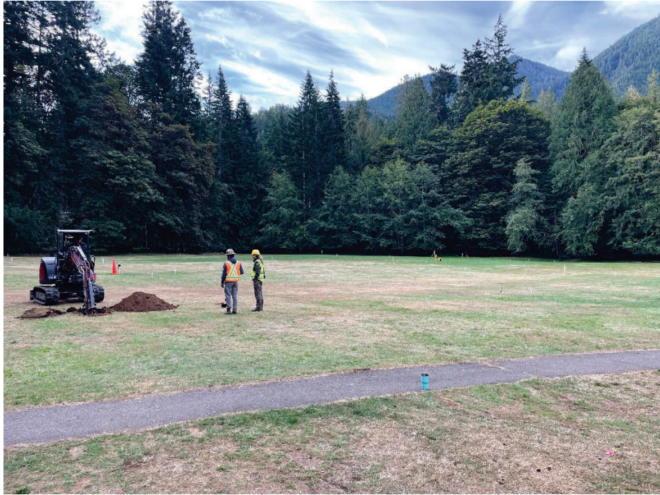
Photograph 7: Recreational field at Lake Crescent Lodge, looking east. The absorption beds are installed under the lawn, within the Lake Crescent Lodge cultural landscape (NPS/2024).
