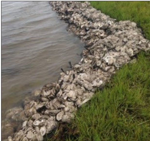
Figure 12. Oyster Bag Revetment
