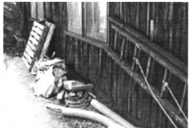
Siding at road level, north side.
