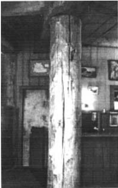
Typical heavy timber column.
