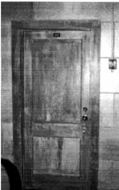
Typical guest room door.
