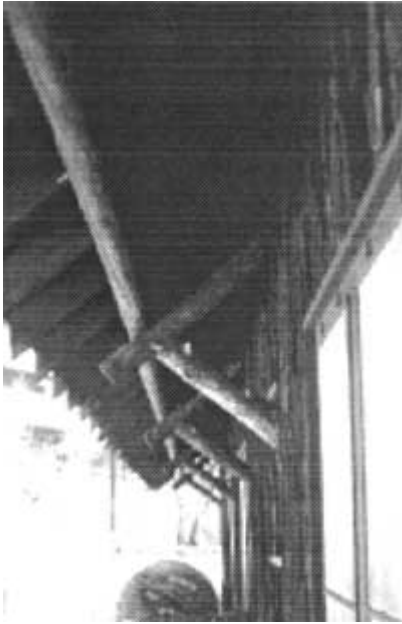
Purlin and brackets, north side.
