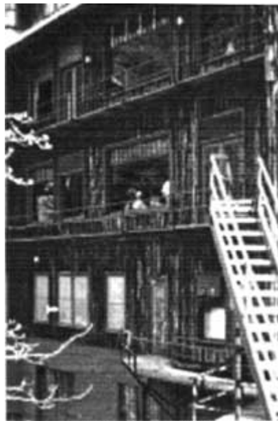
The existing catwalks.
