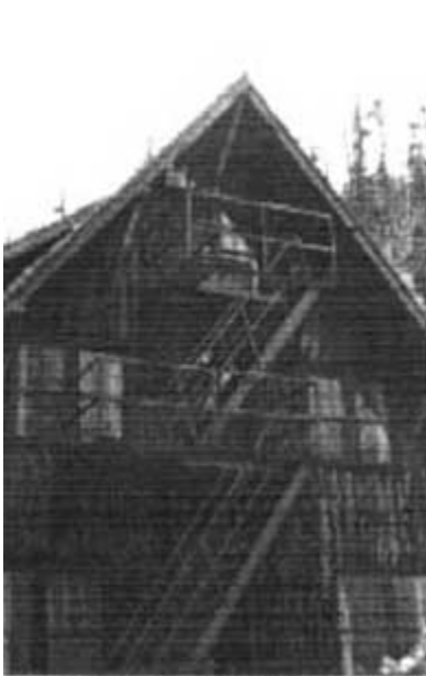
The existing fire escape.
