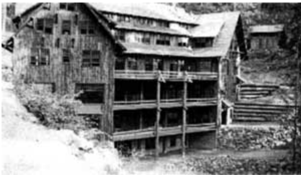
The Chateau just prior to completion. Note that the peeled log and steel fire escapes have not been installed.
