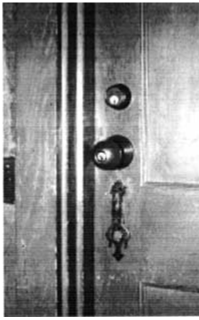
Typical guest room door hardware.
