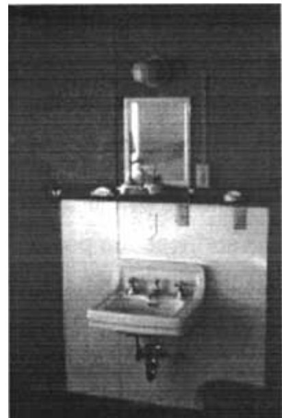
Painted sink surround, 6th floor.
