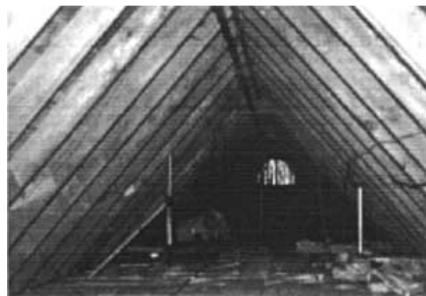
The main attic space.
