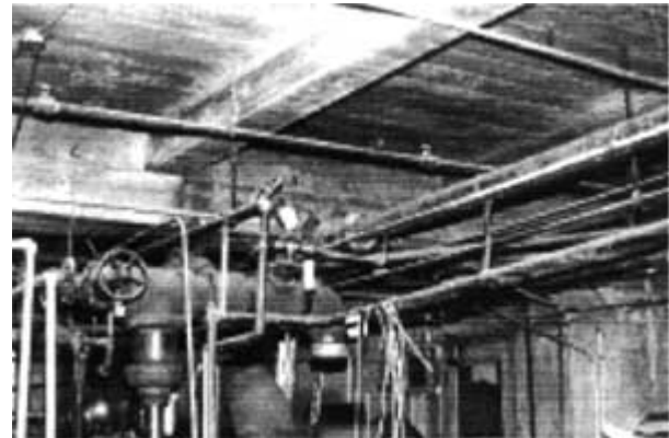
Boiler room ceiling structure.
