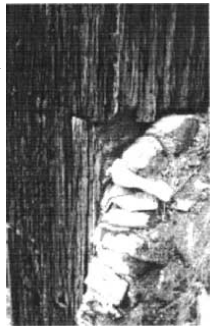
Exposed sheathing at northeast corner.
