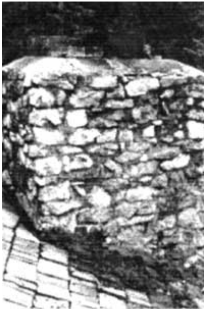
North side of chimney.
