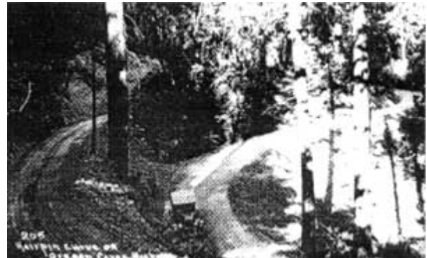
The Oregon Caves Highway, soon after completion.
