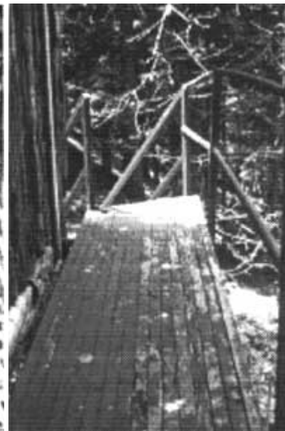
Catwalk pedestrian surface.
