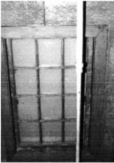
The south attic hatch.
