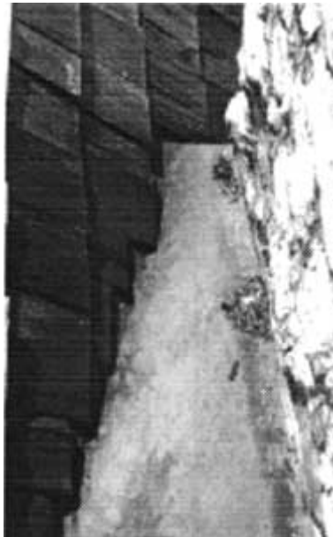
Sheet metal at south end.
