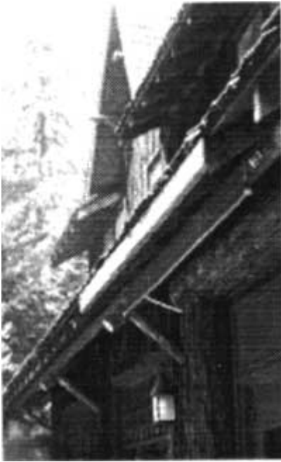
Fascia board for gutter.
