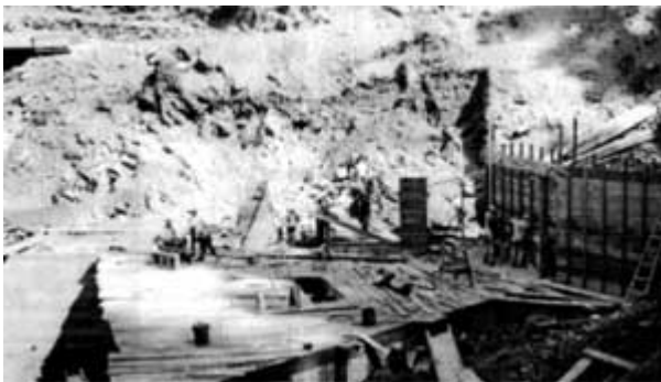
Construction photo showing the concrete forms.
