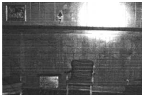
Replacement wainscot in the dining room.
