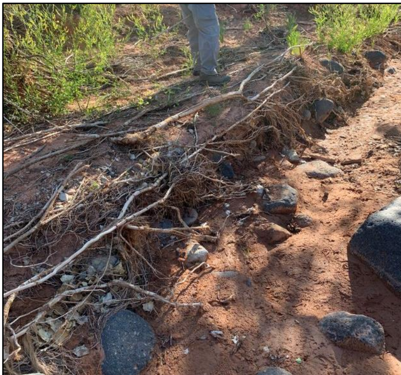
Figure 10. Streambank on Pleasant Creek downstream from the park road. A flash flood in 2022 eroded into the bank, but a strong root network from healthy riparian vegetation limited the erosion and stream widening while preserving a single-threaded channel form with identifiable banks.
