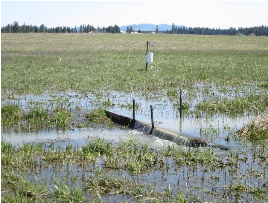
Figure A3. In the foreground a plywood dam causes overbank flows from the ditch that was subsequently permanently filled. In background is the redox station located near Well 12.
