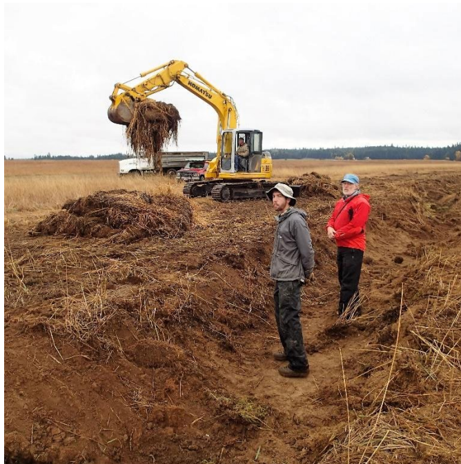
Figure A4: Excavation of ditch and removal of Phalaris arundinacea . Standing around are Derek Schook and David Cooper.
