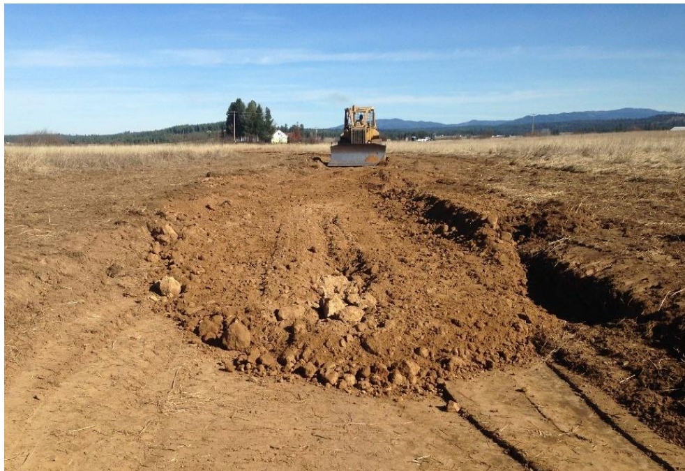
Figure A6. Infilling the ditch. The foreground shows the already filled and compacted ditch, and the weed-free topsoil at center was used for planting.
