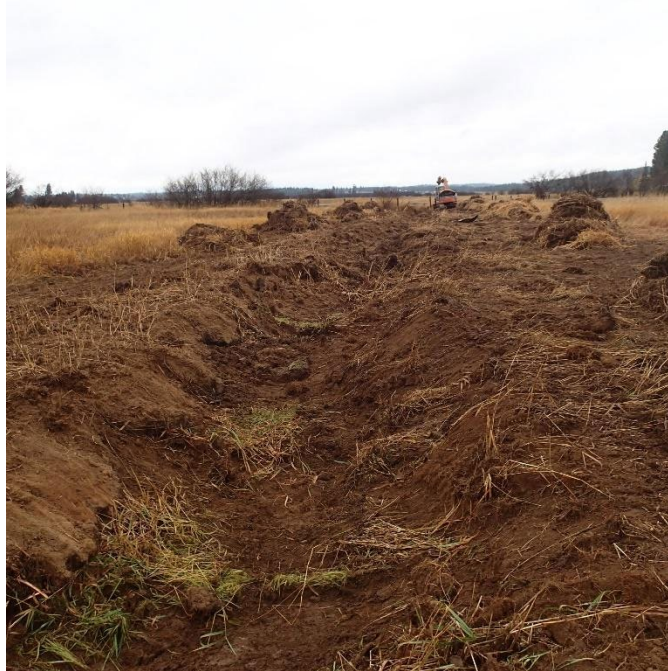
Figure A5: The ditch being excavated, where undercut banks were exposed and Phalaris arundinacea was mechanically removed before infilling occurred.
