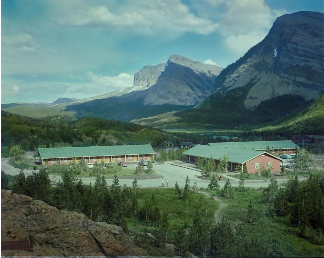
Figure 19. Motel units, Swiftcurrent Motor Inn and Cabins, ca. 1957. The last major expansion of visitor accommodations came in the late 1950s. It featured the motel type of accommodation, popularized by the car culture because motel rooms were cheap and came with private bath and convenient parking. Besides these three units at Swiftcurrent, motel units were added at Rising Sun, Lake McDonald, and Apgar around the same time. (Glacier NP photo, GLAC 10892, Great Northern publicity photo.)
