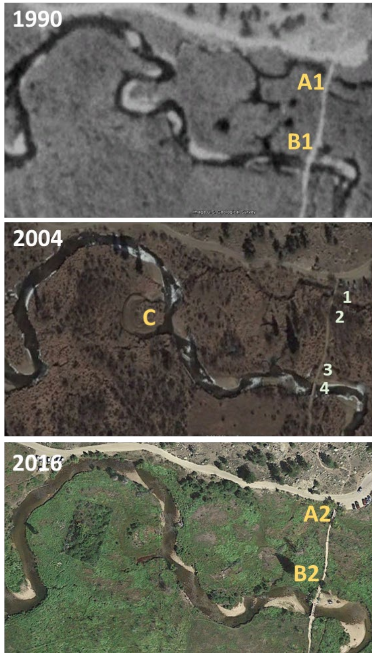
Figure 1. Evolution of the Big Thompson River near the Cub Lake Trail, 1990-2016. The water conveyance structures are labeled in the middle panel and are the small bridge, small culvert, main culvert, and main bridge (1,2,3, and 4). A side-channel that was possibly the former main channel supported surface flow in 1990 (A1) but was completely disconnected by 2016 (A2). The main channel had a relatively straight approach to the bridge in 1990 (B1), but increased sinuosity and a wider active channel developed by 2016 (B2). Increasing sinuosity near the bridge partially resulted from an upstream channel cutoff (C) that steepened the flow gradient and increased energy available downstream. The cut bank at B2 is likely to migrate downstream and compromise the north bridge approach in the future.
