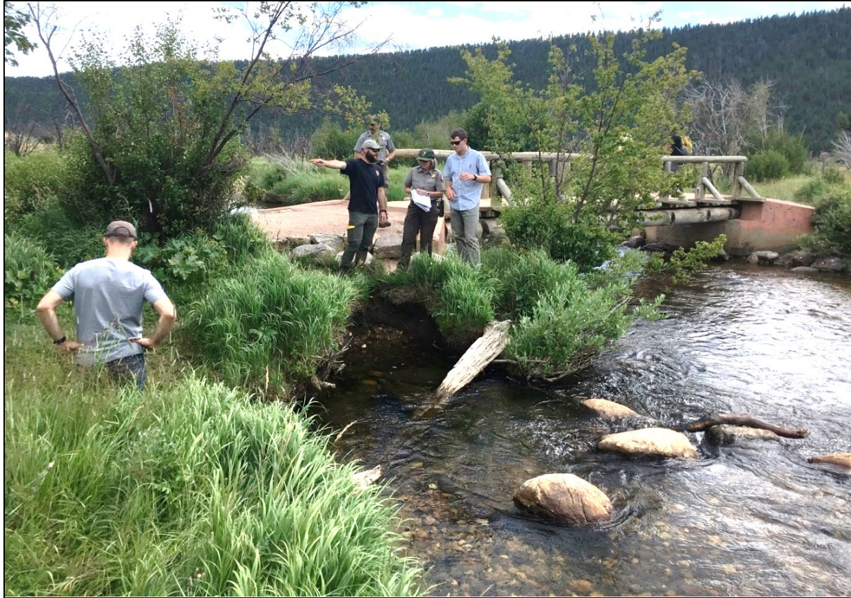
Figure 5. Downstream view of the main channel and its advancing cut bank that threatens the bridge abutment. The small side channel leading to the culvert extends to the left immediately below the researcher at left. This whole section of bank will likely become active channel and be spanned by the proposed boardwalk. NPS, 2019.
