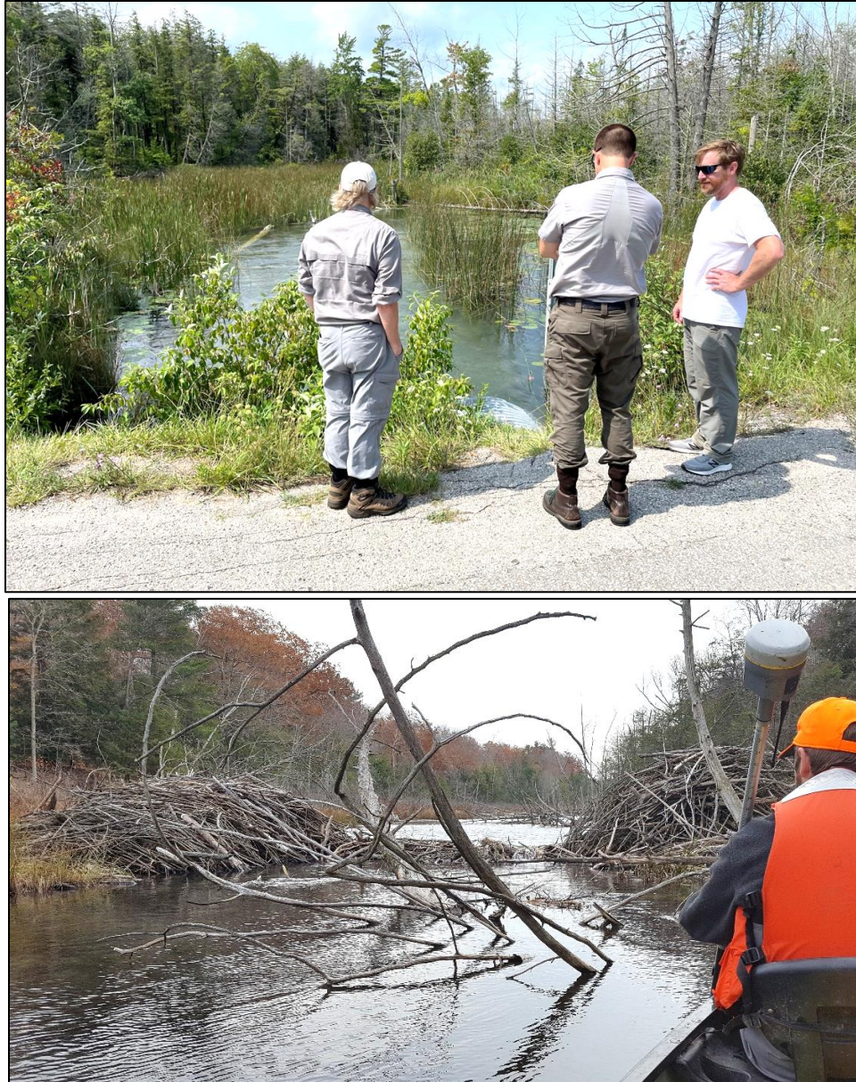
Figure 2. Photos of (top) the downstream view of the existing small arch culvert under West Traverse Lake Road, and (bottom) upstream view of the downstream beaver dam, showing both the dam that backs up water by 0.7 ft and adjacent spoils piles from past breaching events (NPS, 2021).
