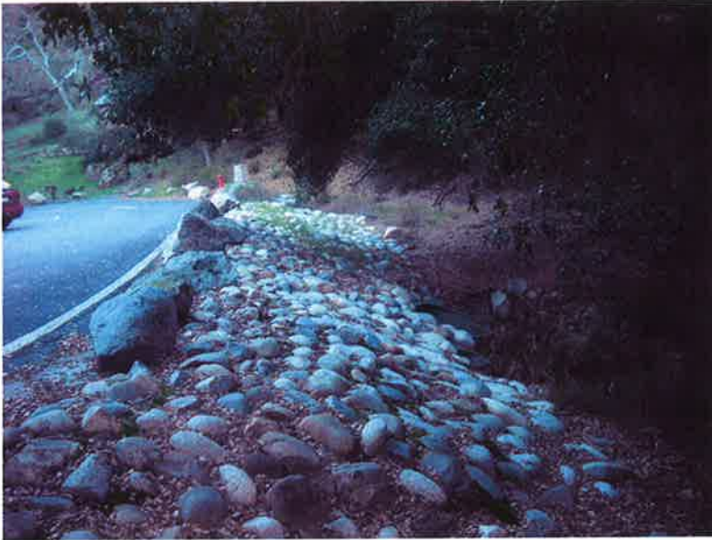
Figure 9. Downstream face of parking lot at Moses Springs
