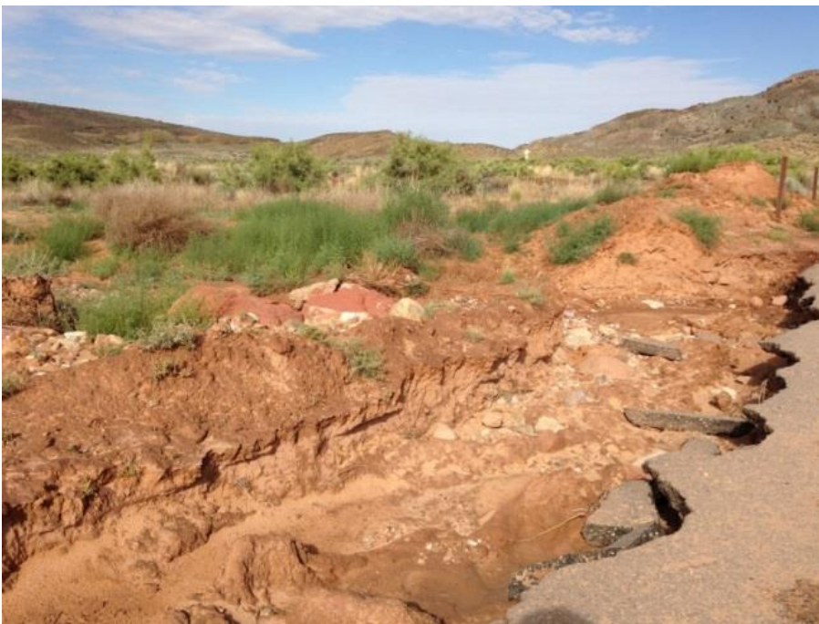
Figure 3. Salt Valley Wash, looking west across the channel from the road crossing. Note the failed asphalt where discharge periodically pours off the road surface. NPS-2016.
