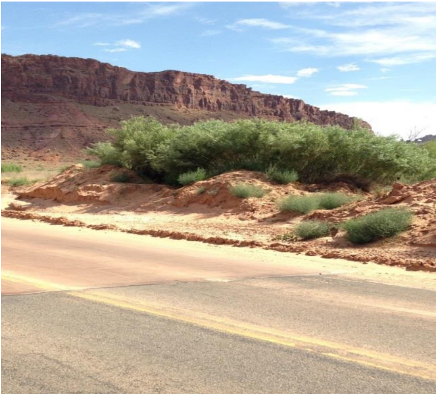
Figure 7. Winter Camp Wash looking down-valley just west of the road crossing. The accumulated sediment is from previous clearing operations and blocks part of a former channel. Note the well-established tamarisk on the mounds of sediment, which are spoil material. The culverts are below grade and completely buried. NPS – 2016.
