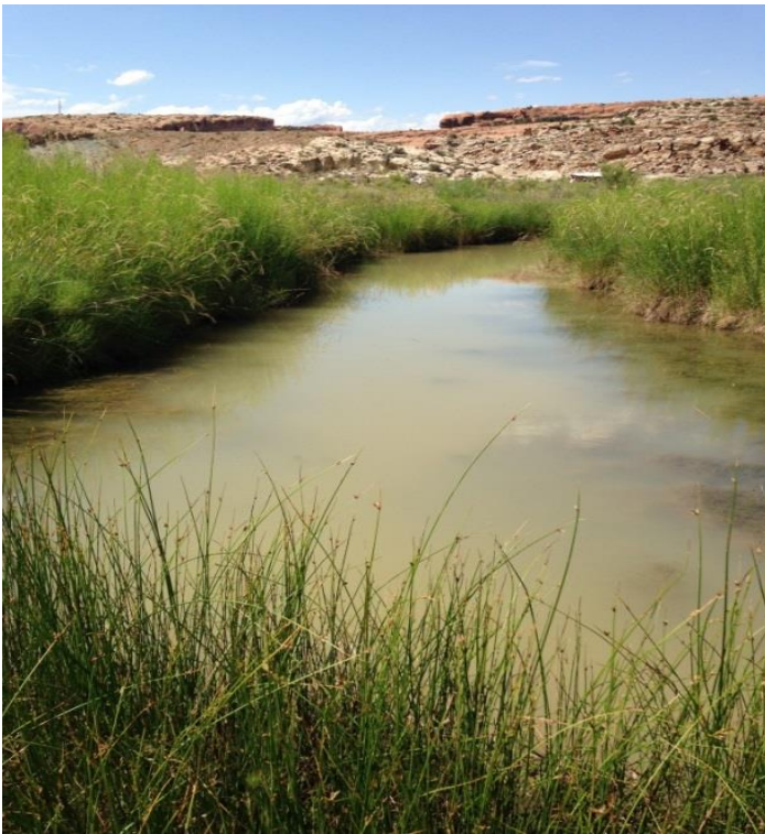
Figure 4. Salt Valley Wash looking upstream from the road crossing. Note that the culvert intake is completely submerged. This channel width may be somewhat representative of historic channel geometry. NPS – 2016.
