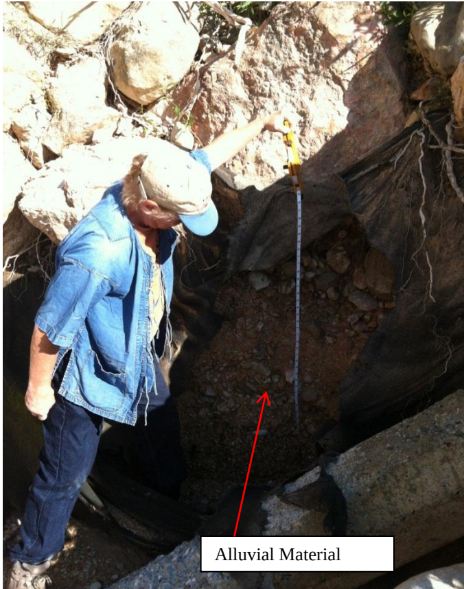
Figure 6 -- About 3.5 feet of alluvial material at the base of the headcut. The dry-stack rip-rap that serves as the base for the concrete drop structure is visible in the upper portion of the picture. Also note the remaining geo fabric that was at the base of the structure. NPS – 2013.
