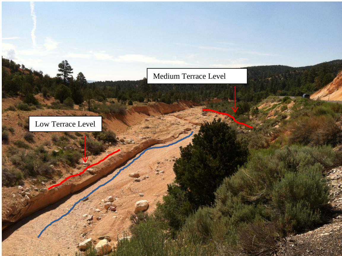
Figure 4 - View of the channel downstream of the drop structure taken from the highway. Note the terrace levels (red lines) and the inner channel (blue line). NPS - 2013.
