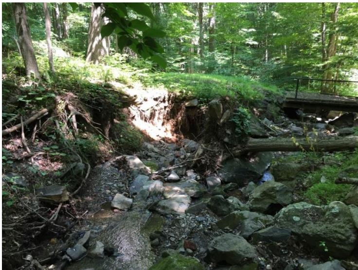
Figure 3 – Incised reach of Ike Smith Stream looking downstream from near the culvert crossing. Note the undercut and fallen trees on the left bank. The vehicle access bridge to the pump house is visible on right side of the image. (NPS-2017)
