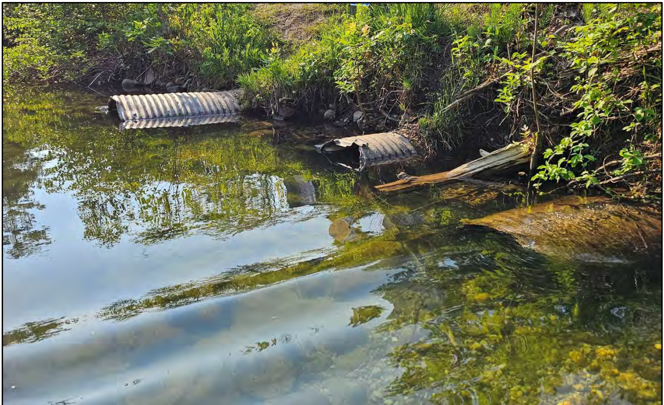
Photo B-30. View of Crossing 2 culverts from upstream, June 9, 2025.
