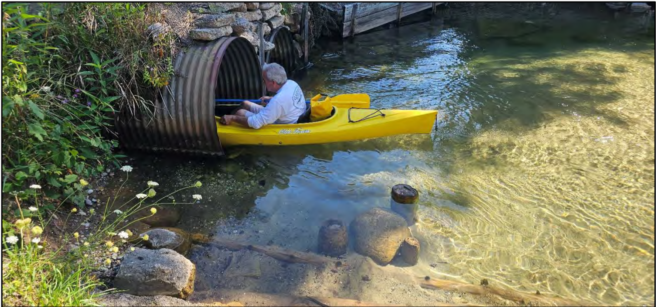
Photo B-2. Additional view of Crossing 3 culvert system with recreational paddler, 2024.
