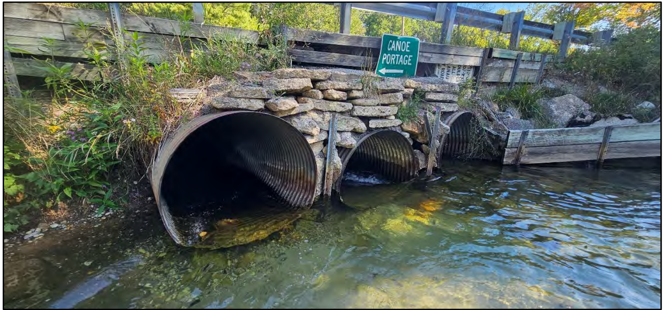
Photo B-1. Photograph of the Crossing 3 culvert system slated for replacement, 2024.
