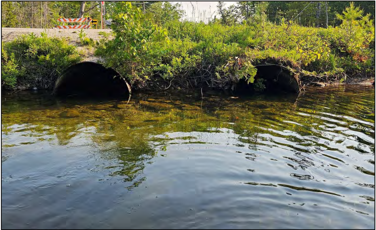
Photo B-19. Upstream view of Crossing 1, June 2025.
