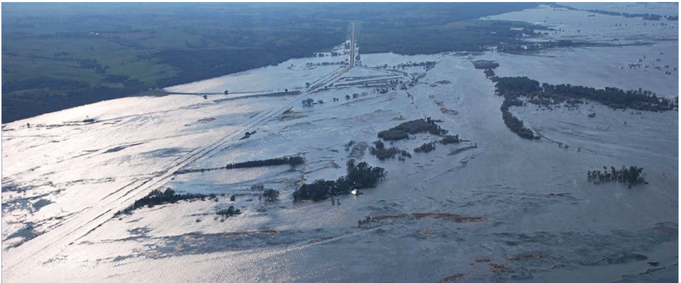
Figure 16. Aerial view of the 2011 flood looking downriver (east) on Nebraska Highway 12. Civil Air Patrol photograph.
