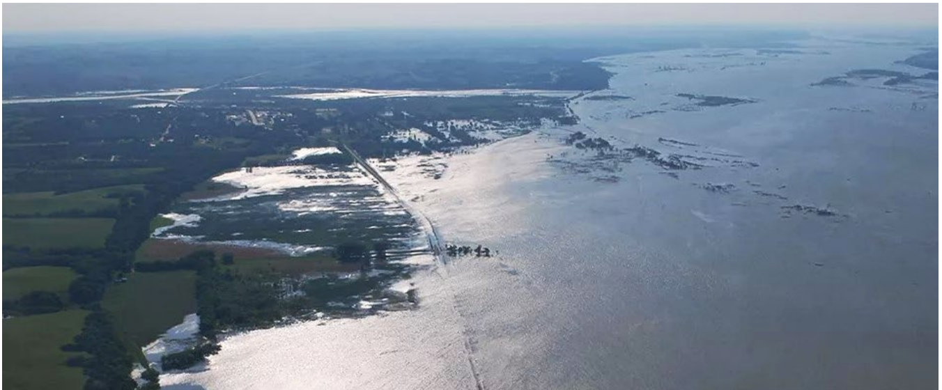
Figure 17. Aerial view of the 2011 flood looking upriver (west) on Nebraska Highway 12 toward the town of Niobrara. Civil Air Patrol photograph.
