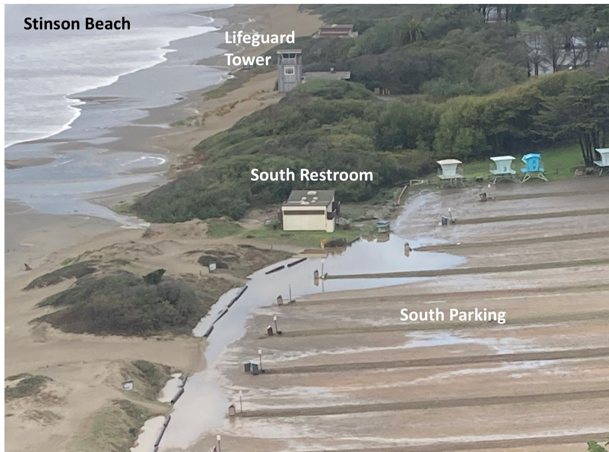
Figure 10. Stinson Beach area, looking north. Note the high water on the beach, dune breaches, and flooding in the South Parking Lot and near the South Restroom. All three of the assets shown (Lifeguard Tower, South Restroom, and South Parking) were reported to be in poor condition and have high sensitivity using this VA protocol. Photo by NPS.
