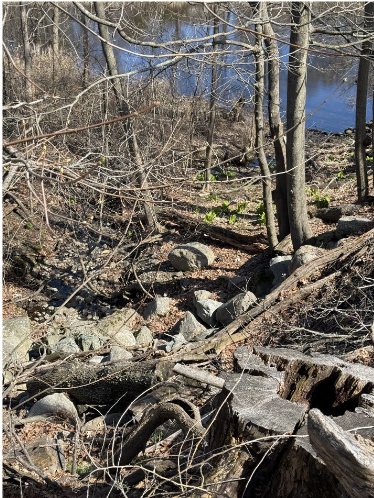
Figure 16. The stone lined channel running down the Forested West Bank area to the Saugus River carries storm water from the parking lot to the Saugus River (NPS, Fuchs, 2022).
