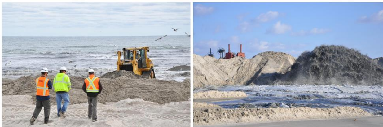
Figure 30. Photos of the winter 2021/2022 construction at Democrat Point. Photographs from USACE.
