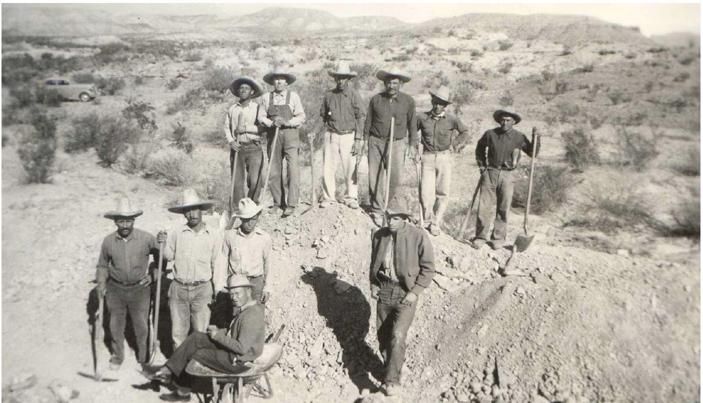
FIGURE 4. Workmen beginning operation at the site of WPA Quarry #1 in Big Bend (Strain, ?1940).
