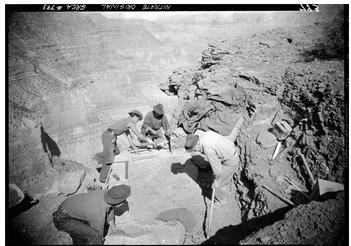
FIGURE 8. CCC workers in 1937 constructing the fossil fern exhibit quarry on the South Kaibab Trail at Grand Canyon National Park (NPS, Grand Canyon Museum Collection, #00793).
