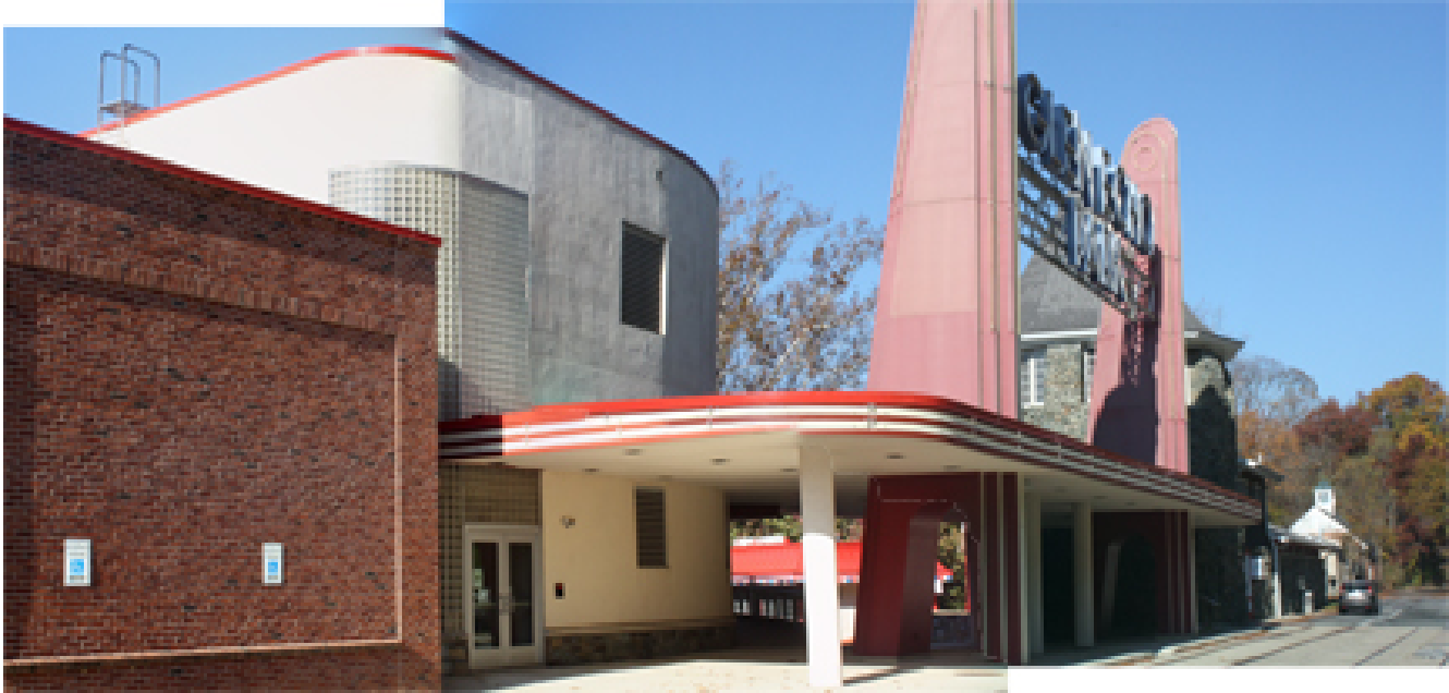
Entrance Portal (NCR CLP 2016).
