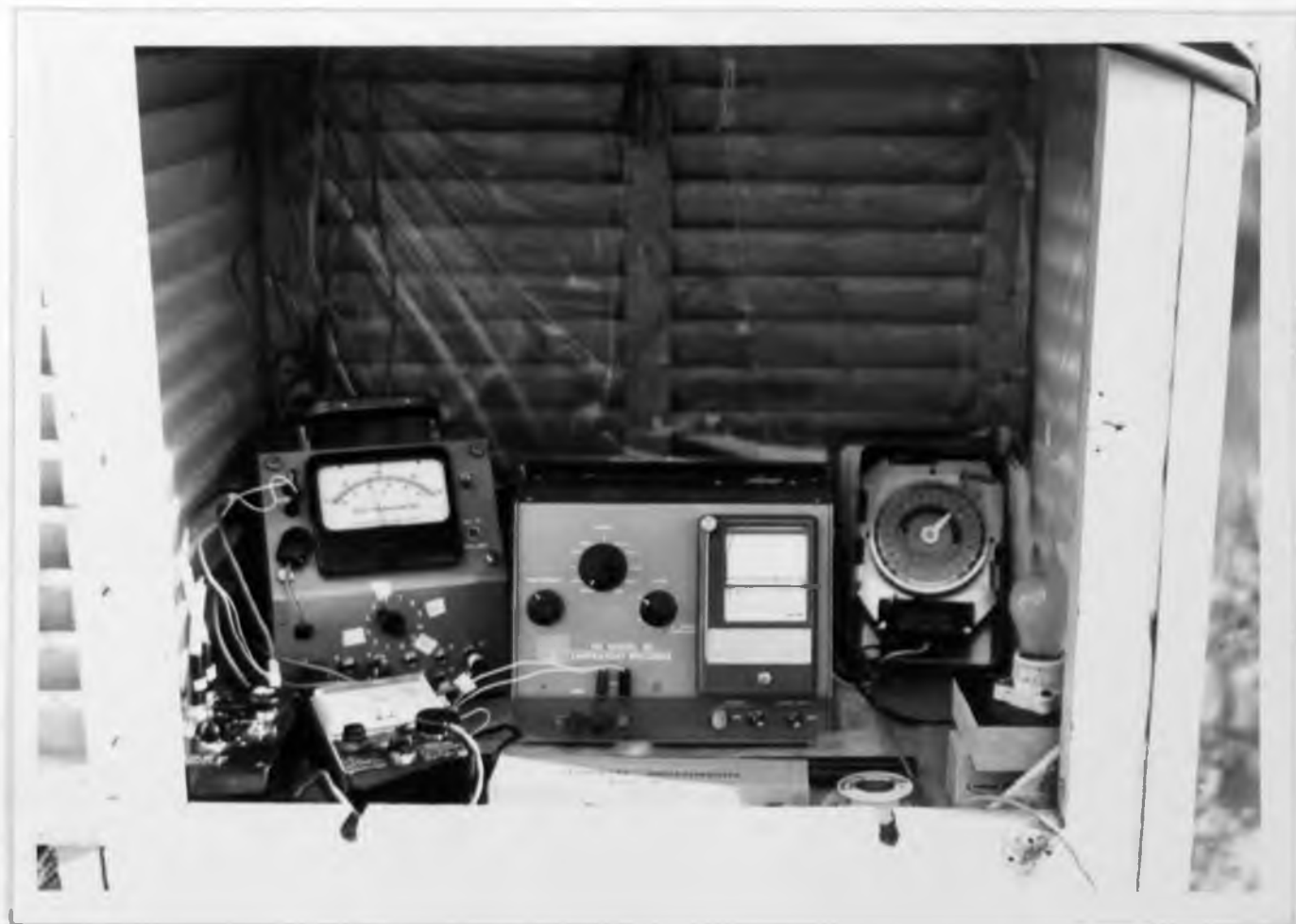
Fig. 2. Interior of the instrument shelter (Fig. 1). Left rear, telethermometer (recorder at center; interval timer at right). Left foreground humidity instrument (junction box and meter).
