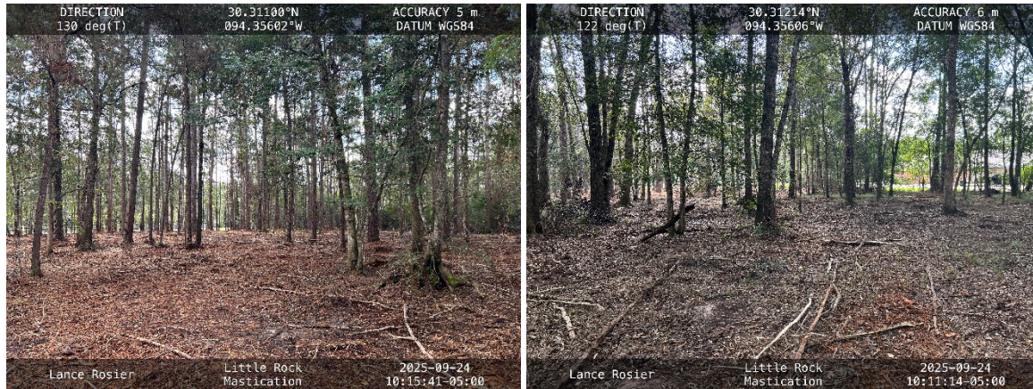
Figure 4. Mastication area behind Little Rock church in Hardin County, TX.
