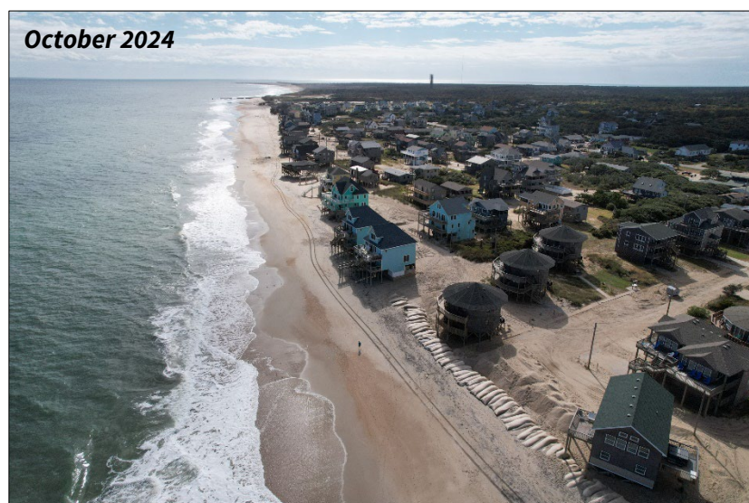
FIGURE 4.9 (page 2 of 6). Before [UPPER], after [MIDDLE], and 2-year post-project [LOWER] images of Reach 1 for the beach nourishment project at Buxton (NC).
