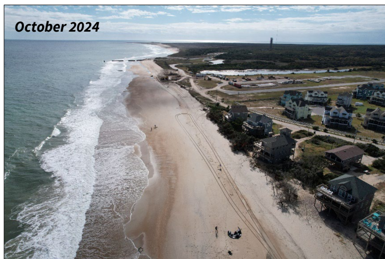
FIGURE 4.9 (page 5 of 6). Before [UPPER], after [MIDDLE], and 2-year post-project [LOWER] images of Reach 1 for the beach nourishment project at Buxton (NC).
