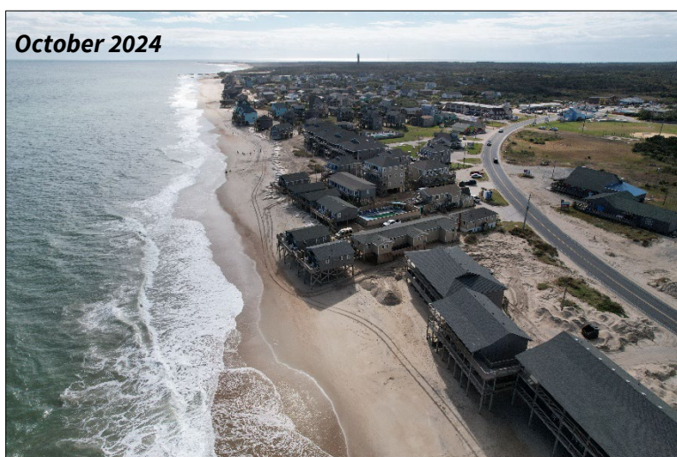
FIGURE 4.9 (page 1 of 6). Before [UPPER], after [MIDDLE], and 2-year post-project [LOWER] images of Reach 1 for the beach nourishment project at Buxton (NC).
