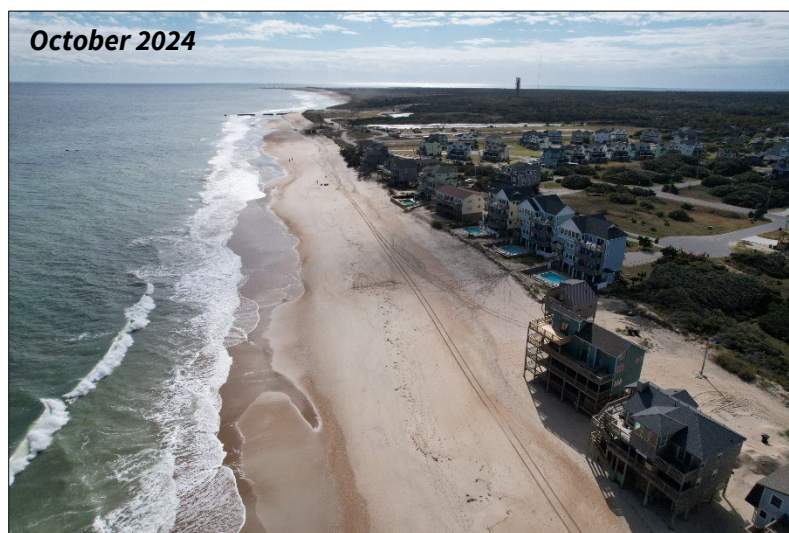
FIGURE 4.9 (page 3 of 6). Before [UPPER], after [MIDDLE], and 2-year post-project [LOWER] images of Reach 1 for the beach nourishment project at Buxton (NC).
