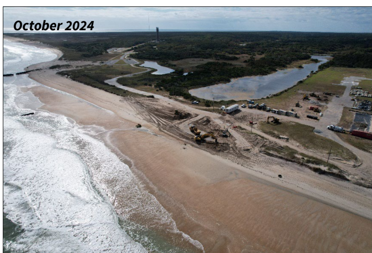
FIGURE 4.9 (page 4 of 6). Before [UPPER], after [MIDDLE], and 2-year post-project [LOWER] images of Reach 1 for the beach nourishment project at Buxton (NC).
