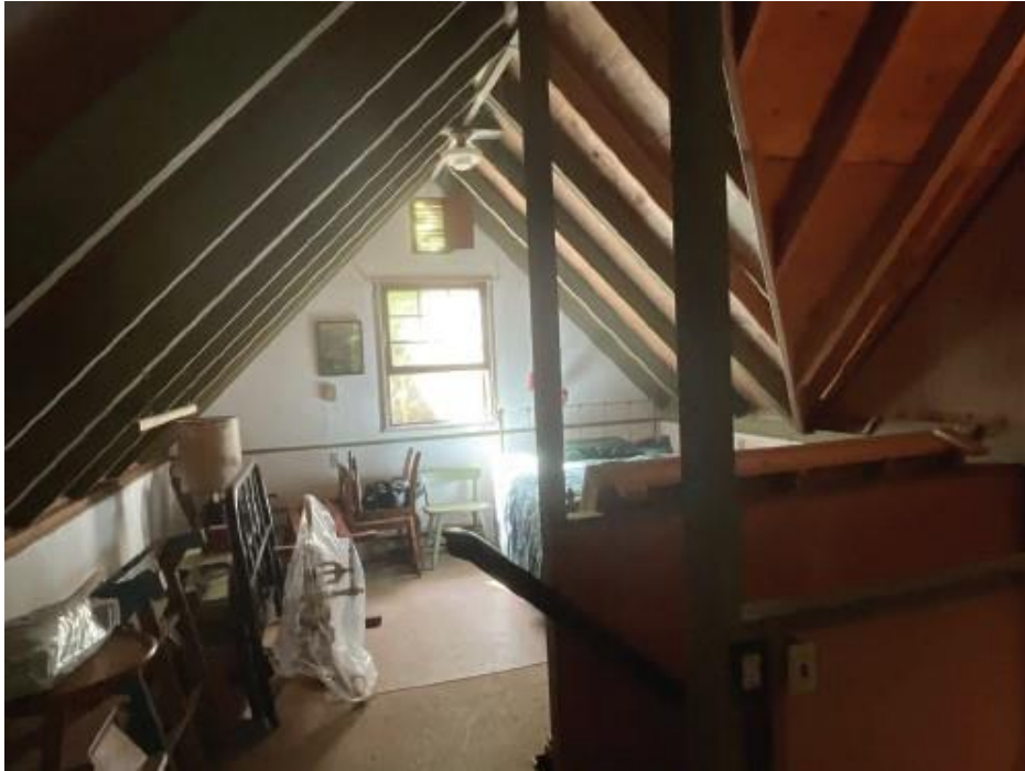
Photograph 11: Interior of loft, showing connection of ell roof to primary gable at photo right, looking south (Deer Park Appraisal, 2024).
