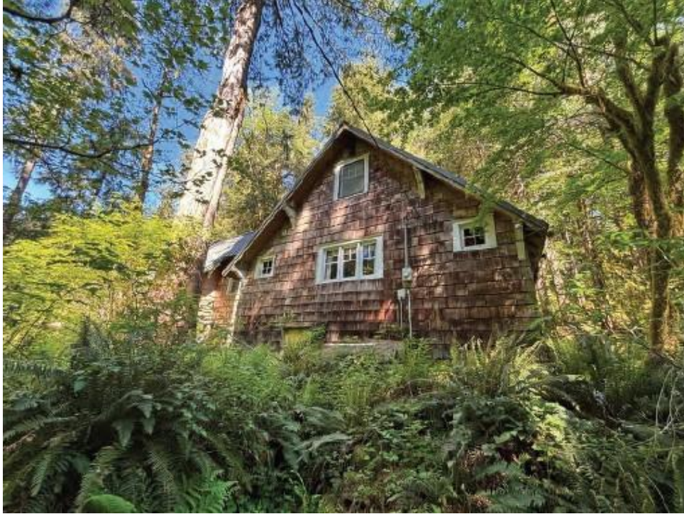
Figure 5: South wall of Webber House, looking north from single car parking space off gravel driveway (Kane Environmental, 2024).
