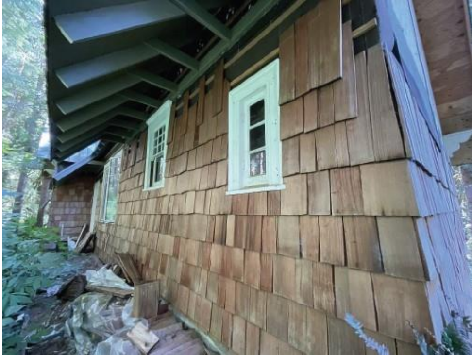
Photograph 7: North wall of ell, looking east toward rear entry and covered stoop (Deer Park Appraisal, 2024).
