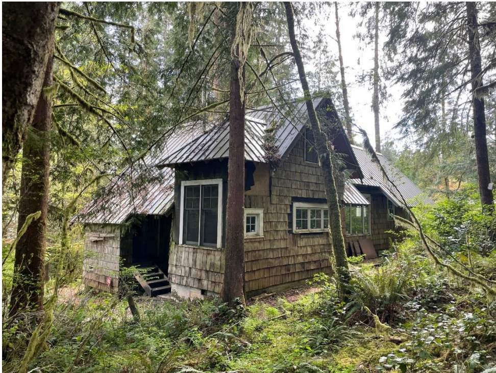
Photograph 8: North and east walls of Webber house, showing corner tower addition, unfinished exterior siding, and enclosed front entry porch, looking southwest (NPS/Matsov, 2025).
