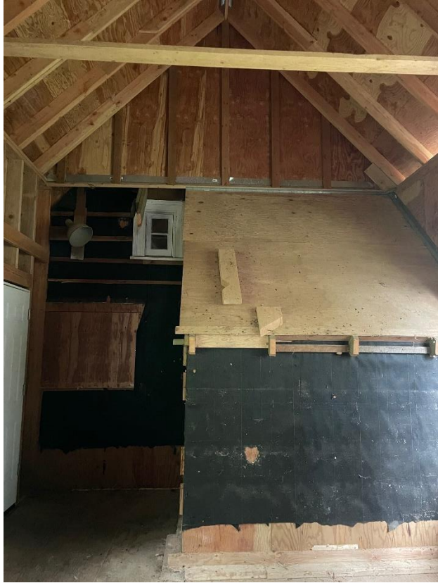
Photograph 13: Interior of ell, showing original west exterior windows and roofline of the house, north exterior door, and unfinished wall and ceiling configuration (NPS/Matsov, 2025).
