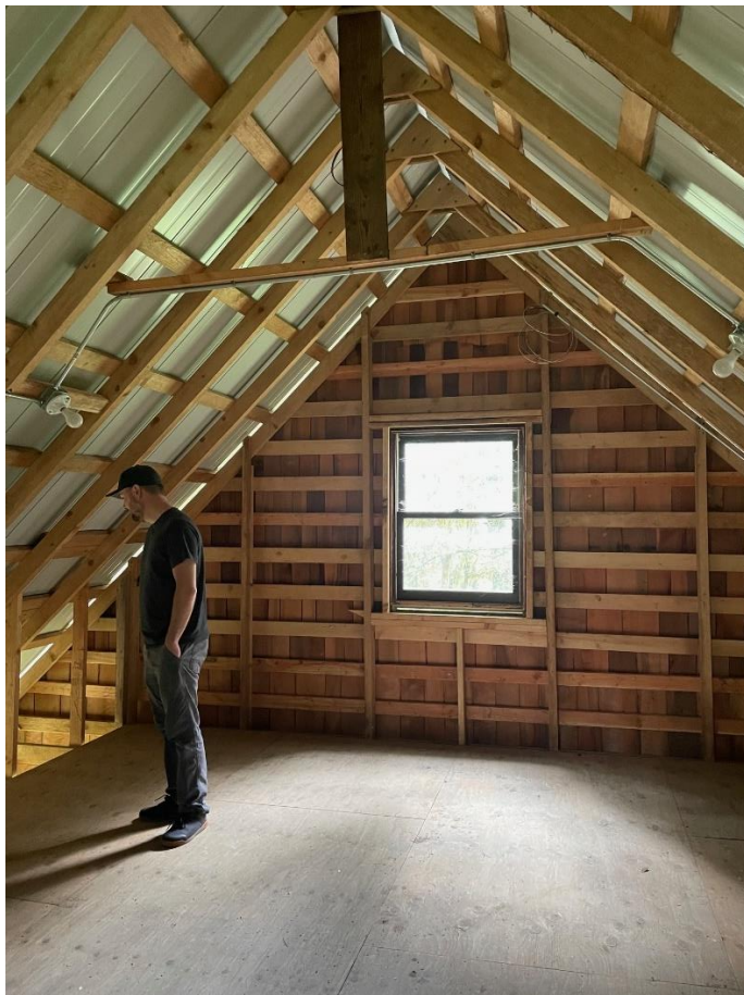
Photograph 16: Interior of carport loft, looking west (NPS/Matsov, 2025).
