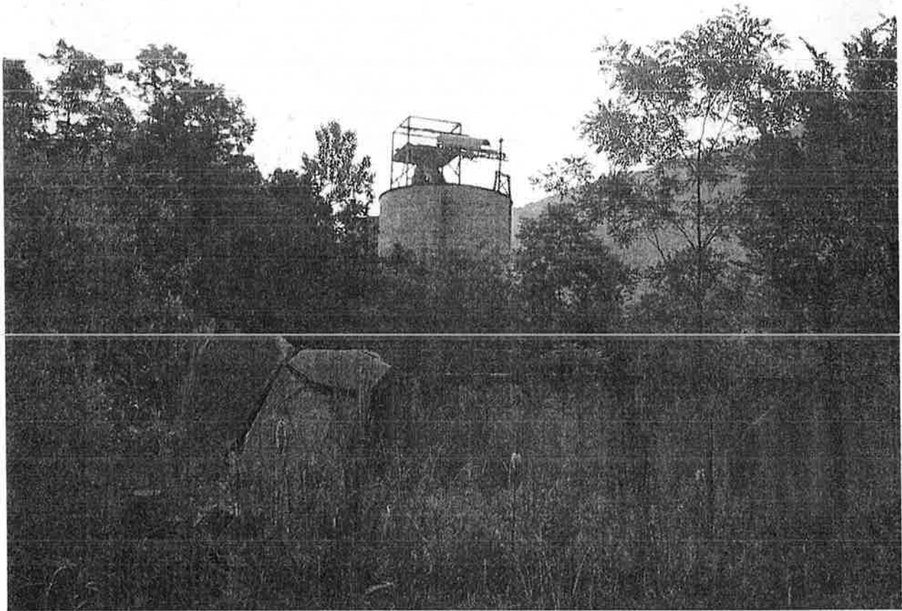
Figure 12: Concrete silo and thickener at Royal Coal Company IHTIA, 2003
