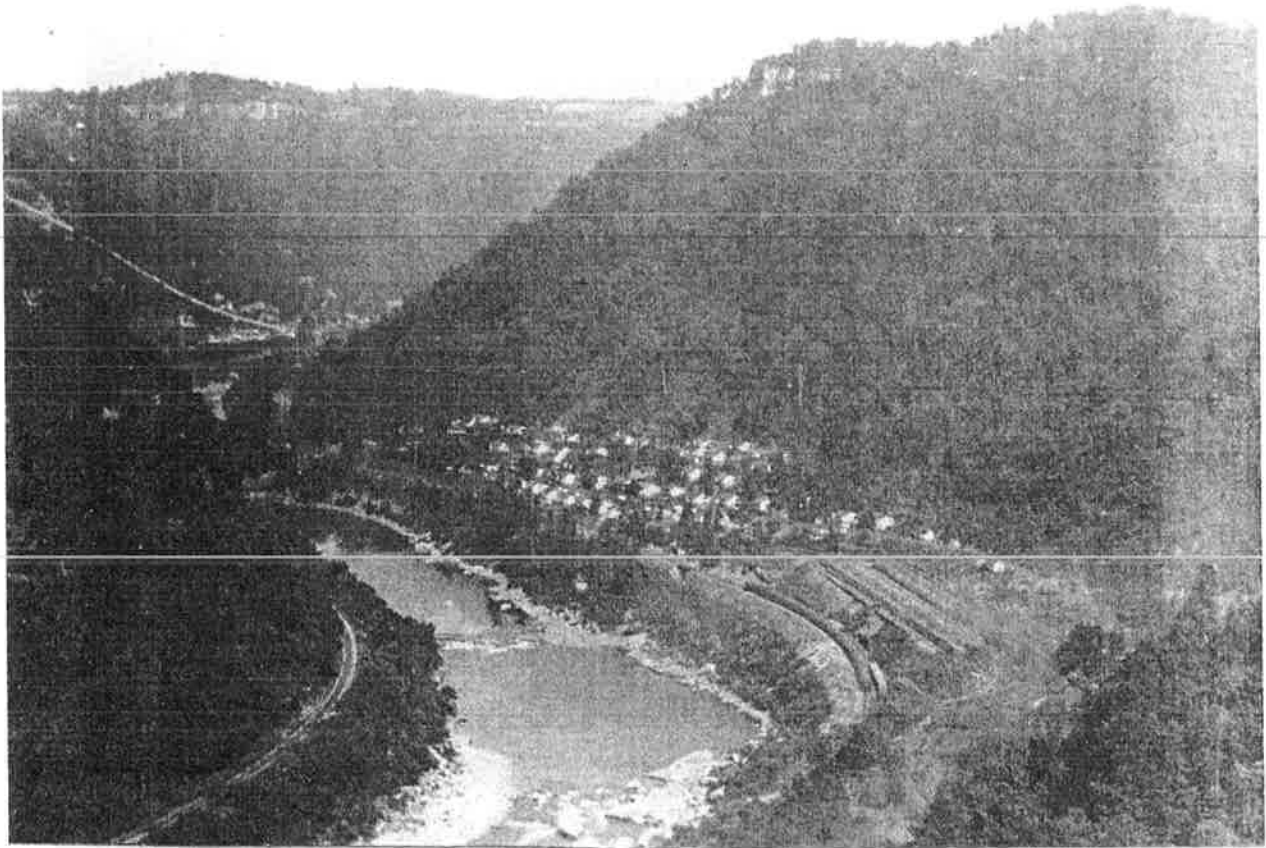
Figure 25: Kay Moor Bottom looking south with Nuttallburg conveyer at upper left NERI Historical Collection
