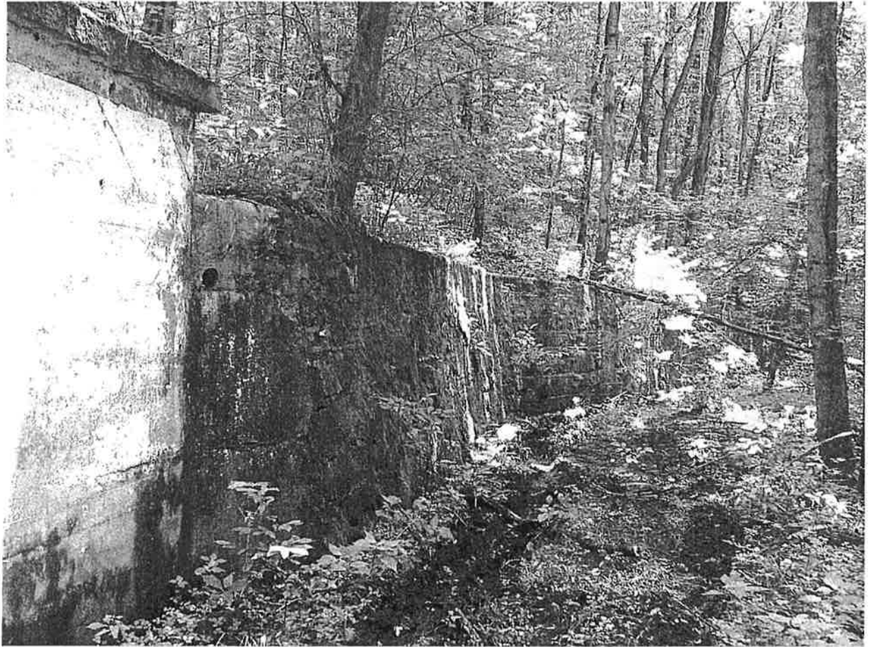
Figure 19: Stone walls at McKendree IHTIA, 2003
