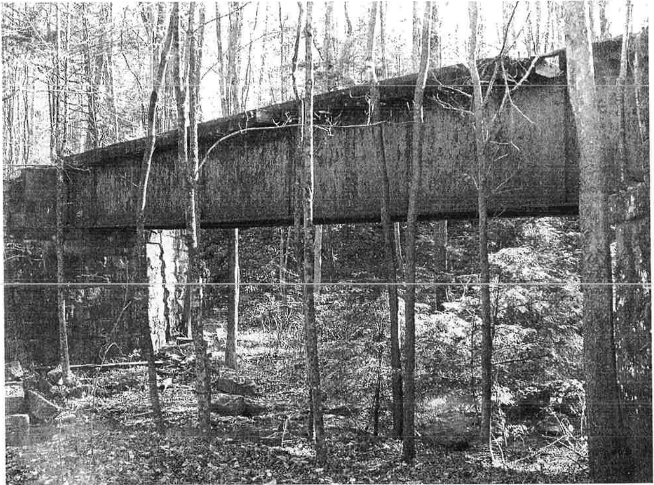
Figure 40: Steel plate girder bridge on Keeney's Creek IHTIA, 2003
