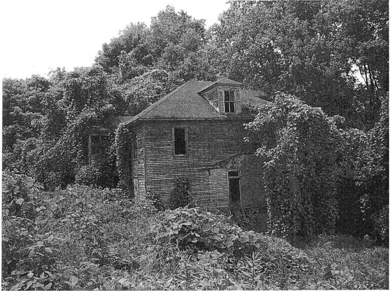
Figure 17: Former boarding house at Thayer off State Route 25 IHTIA, 2003
