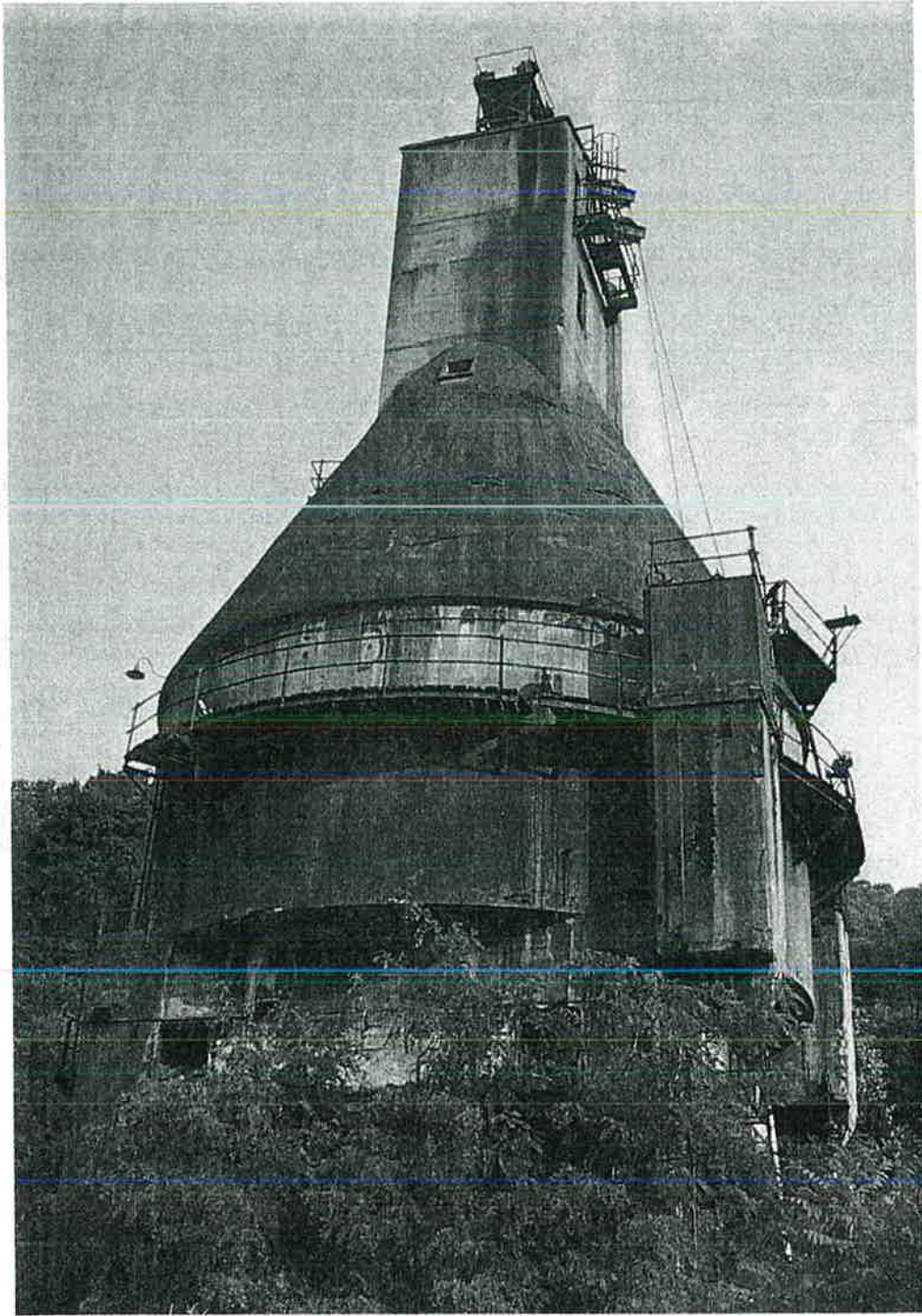
Figure 38: Concrete Coaling Tower at Hinton IHTIA, 2003
