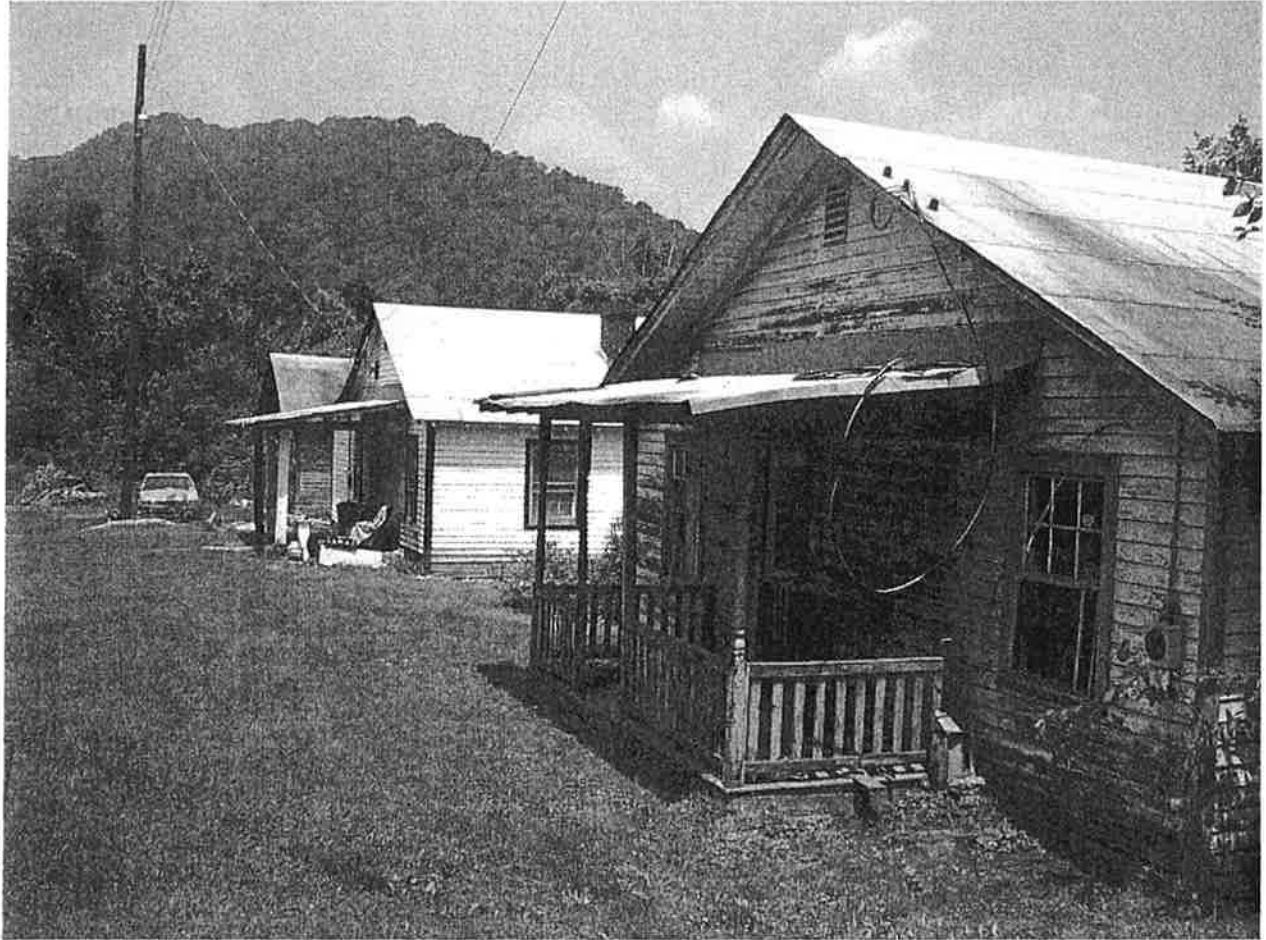
Figure 15: Former miner's houses at Thayer off State Route 25 IHTIA, 2003
