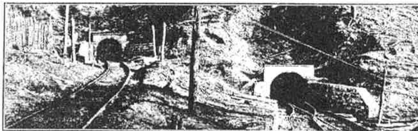
Masonry Mine Portal
