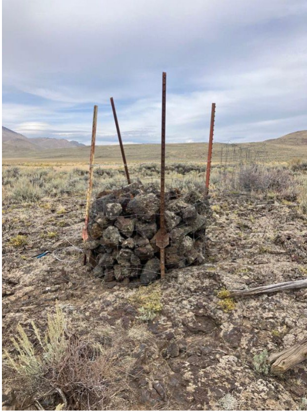
(Left) Rock crib constructed when t-post could not be pounded into ground. Crew used the rock crib to stretch wire over the lava rock; (right) Megan Bench and Amanda Voth clip and nail in new smooth wire (9/29/23).
