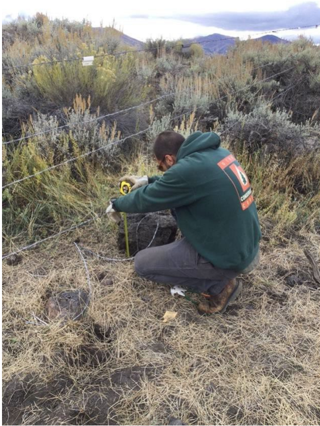
Kody Kitchener (left and right) installing a rock hang that brings down the fence height to the proper eighteen inches (43.534591, -113.526592).
