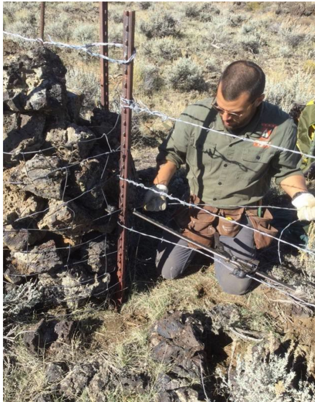
(Left) Member Kody Kitchener tying off a wire to a rock crib after stretching it (43.534551, -113.529980). (Right) Section of nearly finished fence leading to a rock crib (43.534861, -113.531903).
