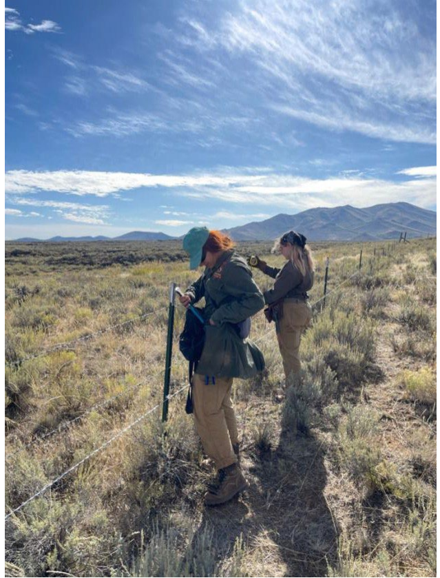
(Left) Rock crib constructed when t-post could not be pounded into ground. Crew used the rock crib to stretch wire over the lava rock; (right) Megan Bench and Amanda Voth clip and nail in new smooth wire (9/29/23).
