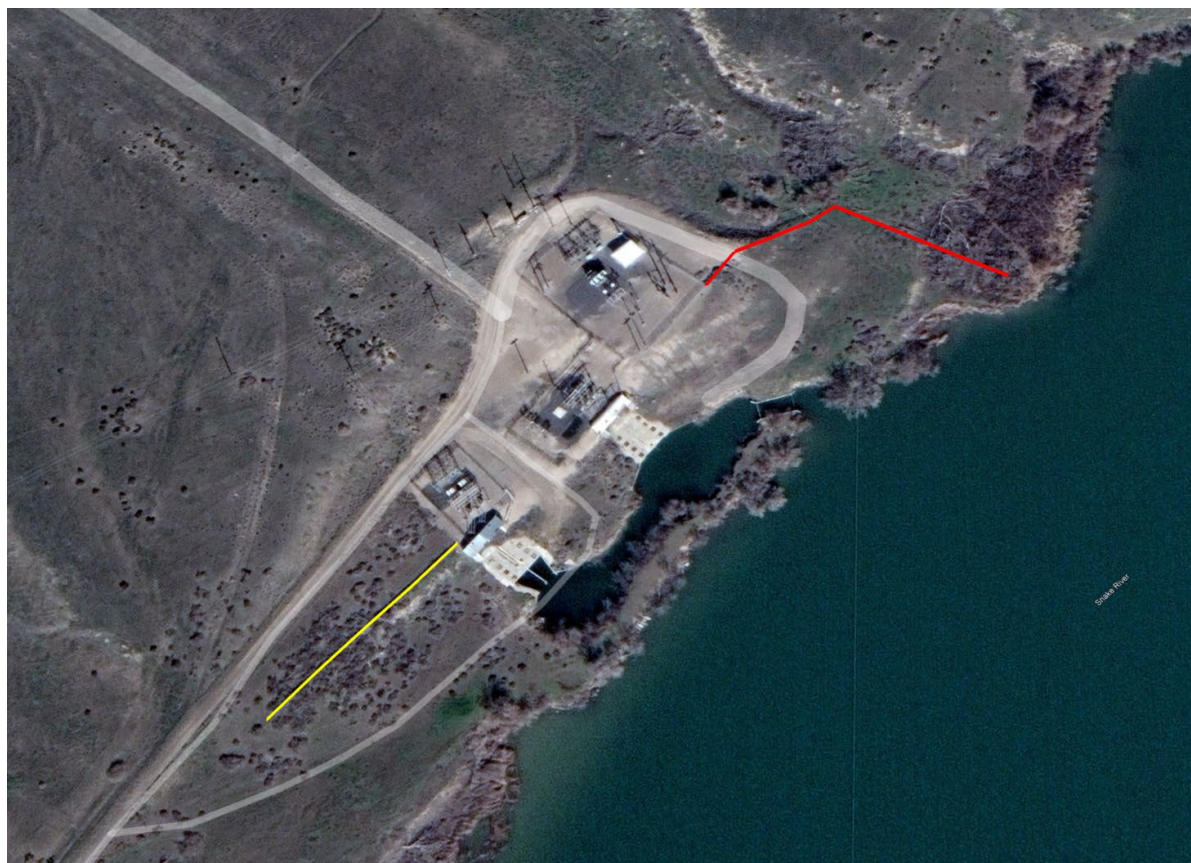
Hagerman Fossil Beds: Fence around the Fossil Gulch substation. Red=312 feet of barbwire fence removed. Yellow = 213 feet of post and rail with barb wires on it removed.
