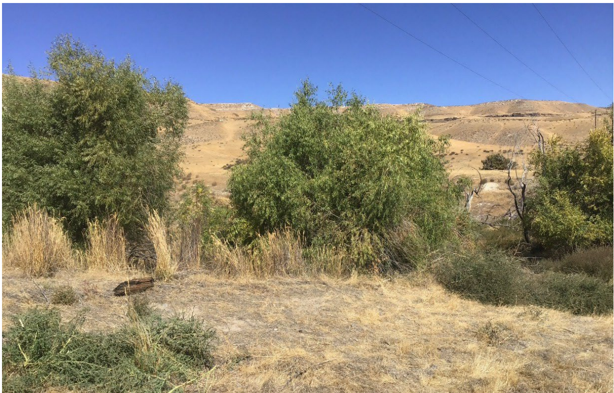
HAFO: Fence removal by UCC crew.
