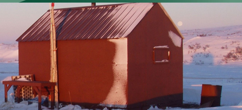
Aniagaaq Ranger Station – Cape Krusenstern National Monument. NPS Photo
