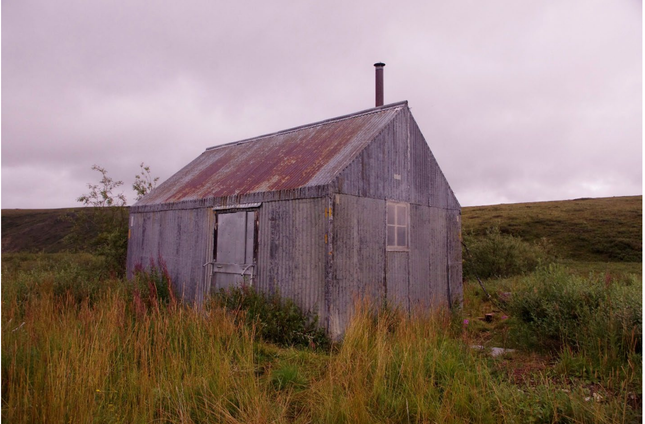
Photo 4: Cottonwood Shelter Cabin, Southwest, NPS Grant Crosby, 2023
