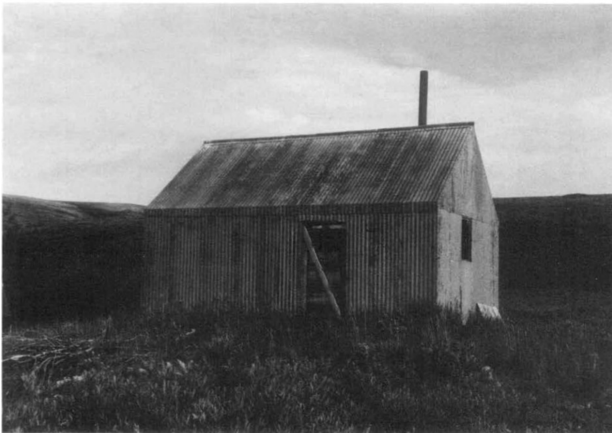
Figure 3. Cottonwood Shelter Cabin, 1985. NPS photo by Frank Williss.
