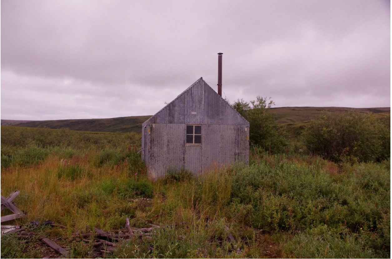
Photo 5: Cottonwood Shelter Cabin, Southeast, NPS Grant Crosby, 2023
