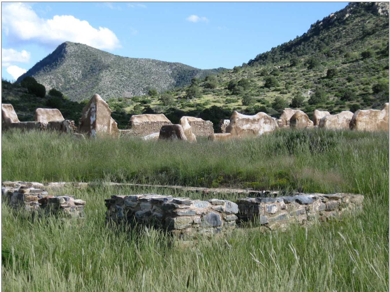
Bath house and laundry room—Fort Bowie National Historic Site.
