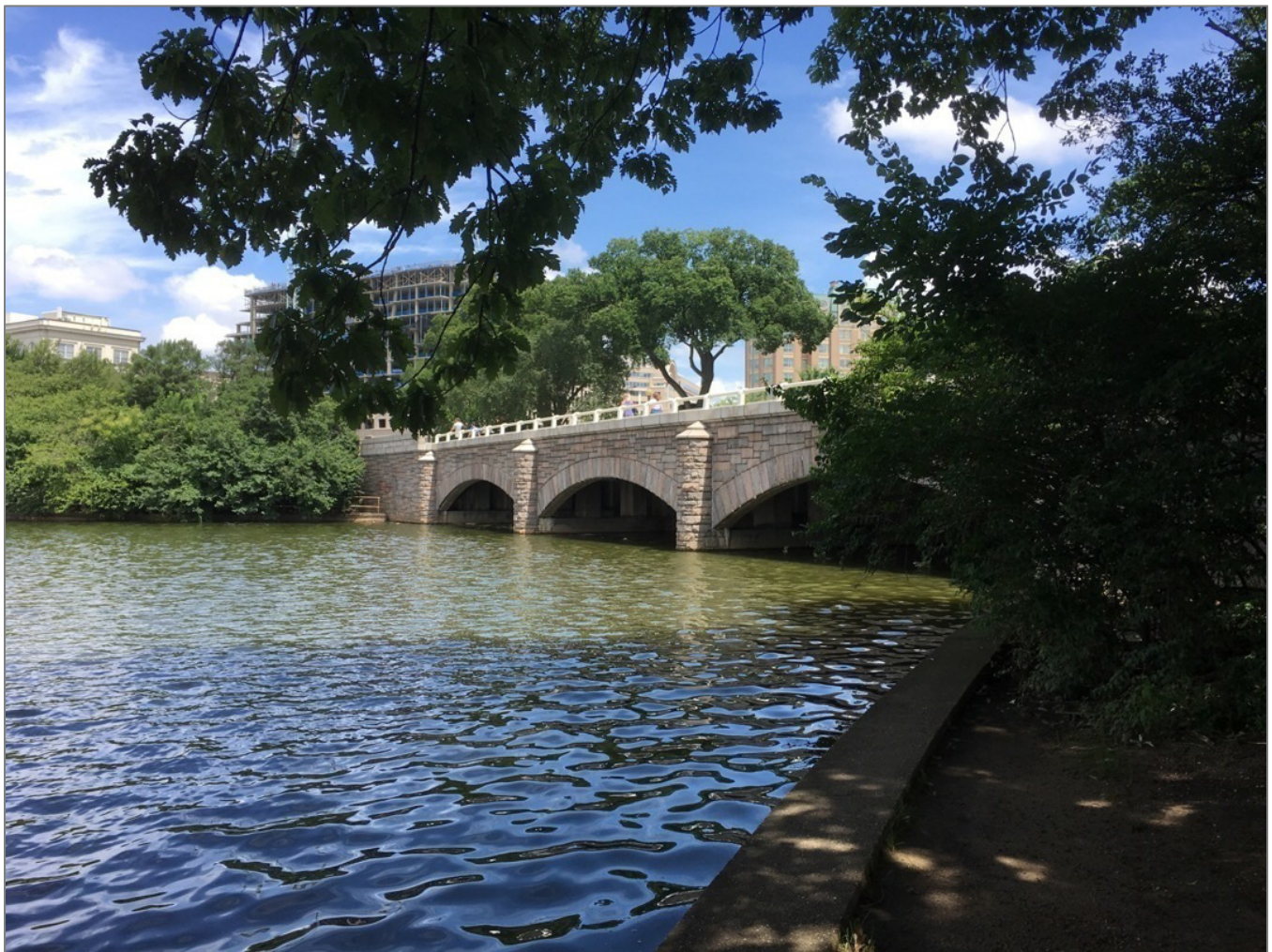
Outlet Bridge spanning the Tidal Basin.
