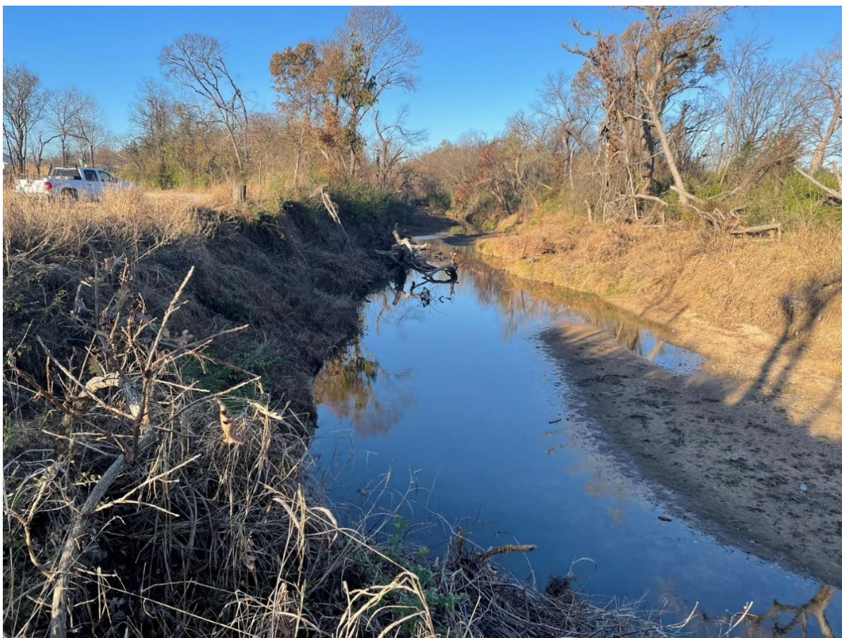
Figure 3. Upstream view of Rock Creek near Black Sulphur Springs picnic area. The channel bank at left has recently eroded, but the straight reach, the non-vertical bank, and quick revegetation suggest that further bank erosion will not extend significantly into the picnic area.
