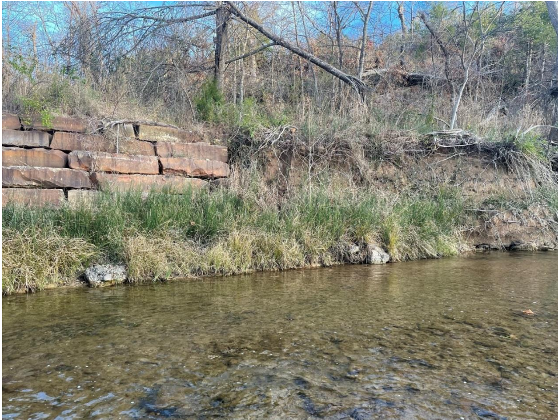
Figure 5. The rock revetment wall on Rock Creek just downstream from Job Corps Bridge. Note 1) sedimentation with subsequent plant growth now stabilizes its base, 2) no flanking or excessive erosion on its downstream (right) end, and 3) living and downed vegetation are present to protect the bank and overbank areas during floods.
