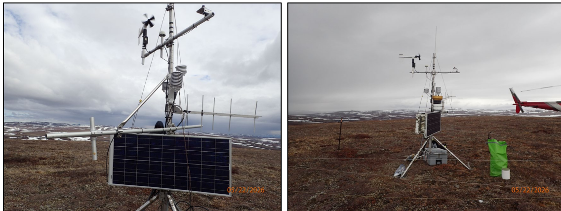
Figure 14. Tahinichok climate station with missing rain gauge (left) and after site visit (right) on May 22, 2026.
