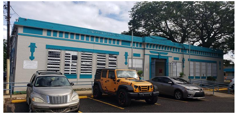
Schoolhouse' front elevation, looking northeast. Photo by Luis René Rivera
