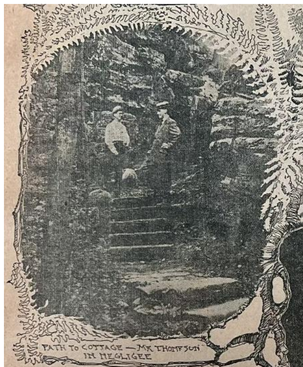
Figure 5. James Thompson and J.M. Megligee on stone steps. This 1906 photo is from Reference 3.
