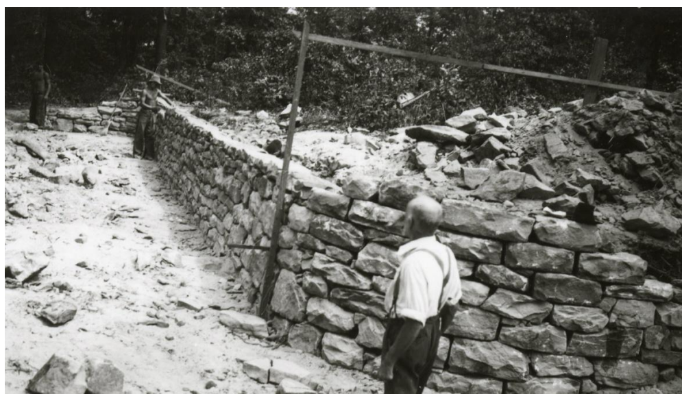
Figure 15. Retaining wall being built by the CCC in August 1934, near the site of James and Edna Thompson's Stone House. Courtesy: Summit Metro Parks.
