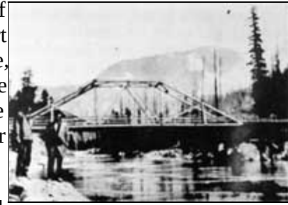
First Bridge Across Middle Fork
