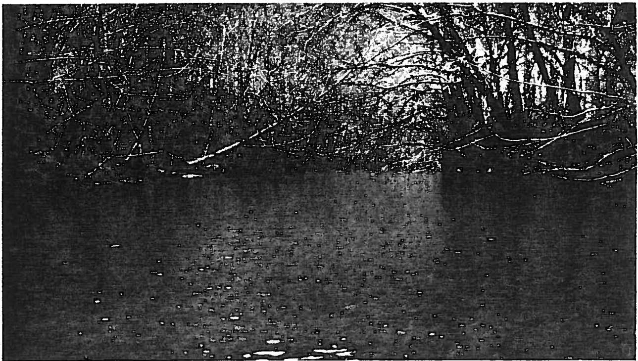
View upstream from top of the dam.
