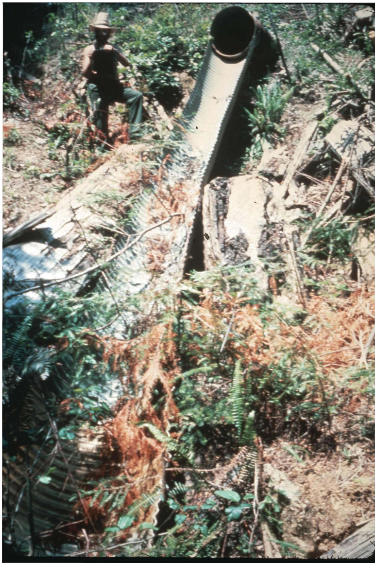
Unit: 82-4 Ref. 2-A 6/16/82 PP#34 Fill Slope RX 14 G.B.
