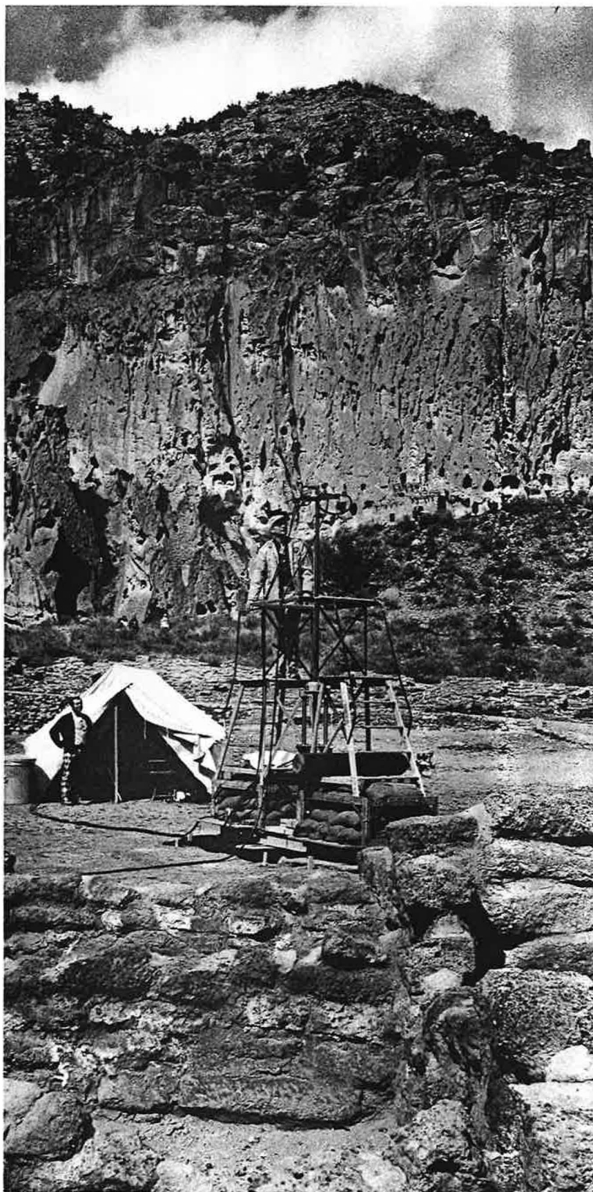
Olivas checks melting rate by viewing measuring stick on stem of subterrene through telescope.
