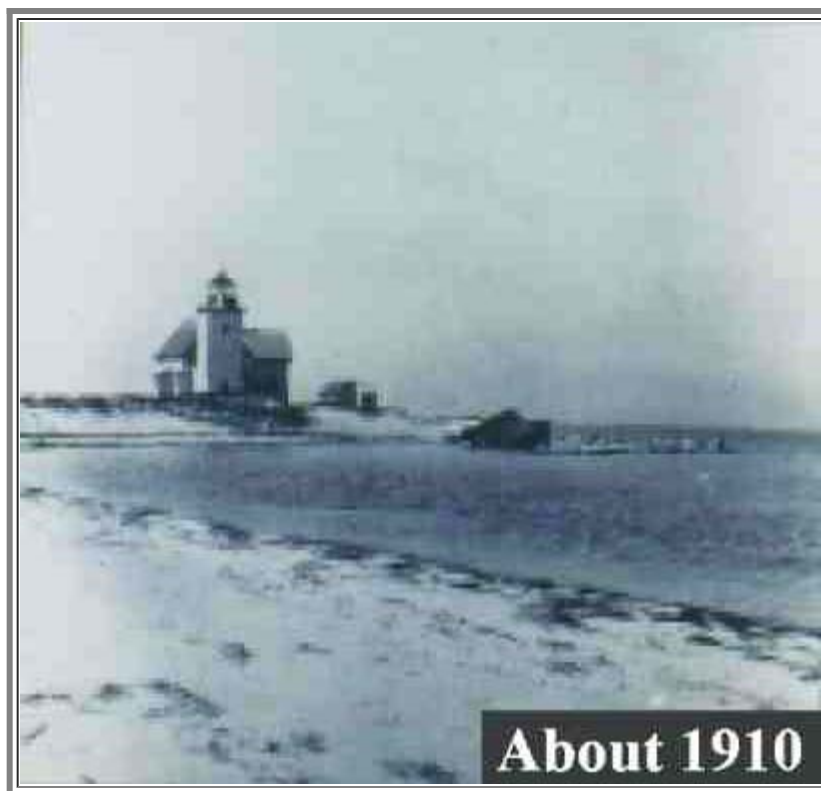
Figure 26. Billingsgate Island before the entire island was eroded away. It is clear that shore erosion is threatening the lighthouse as the sea wall of boulders was built in a futile effort to protect the lighthouse from wave attack. Unfortunately, the sea wall was poorly placed and actually increased the rate of erosion (photo provided by the Cape Cod National Seashore).
