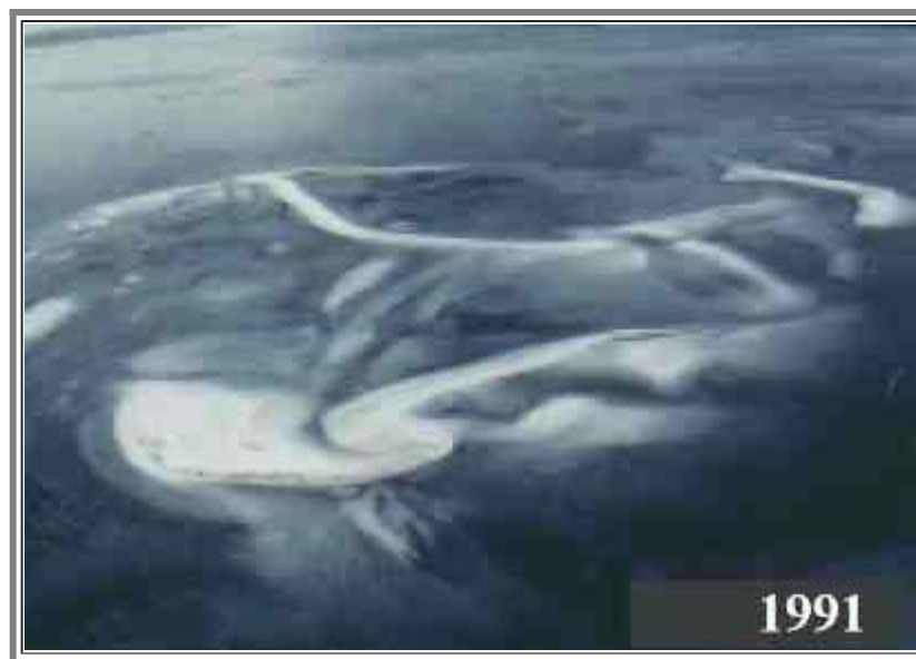
Figure 27. The remains of Billingsgate Island of Wellfleet. Photographed at about low tide in 1991. Today all that remains of the island is a shoal exposed during very low tides. Blocks of stone behind the boulders of the original riprap sea wall are all that remain of Billingsgate lighthouse. The fate of Billingsgate Island may be a precursor for Cape Cod as the sea continues to erode the fragile land (photo by Dann S. Blackwood, U.S. Geological Survey).
