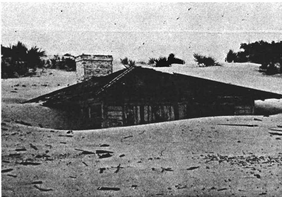
Figure G-18. This house was built west of the back dunes. Subsequent dune migration covered the house and it is now emerging on the east side of the dunes. Nightingale Avenue, Cumberland Island.
