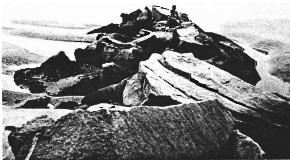
Figure G-10. The jetty located on the south end of Cumberland Island is acting as a sediment trap causing growth of the island.
