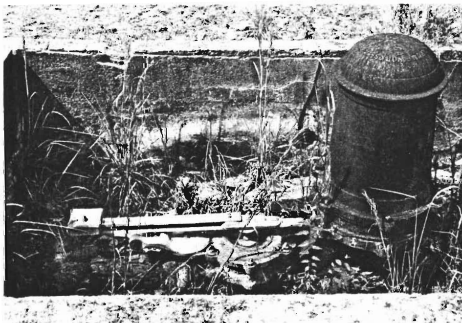
• Figure G-20. Hydraulic ram used to pump water without electricity, Dungeness, Cumberland Island.
