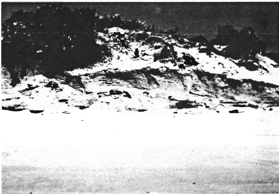
Figure G-14. Close up of dune erosion resulting from Hurricane David.
