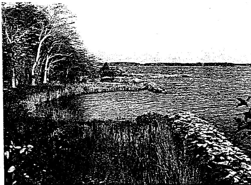
Stone sill and breakwater project after 5 years.
