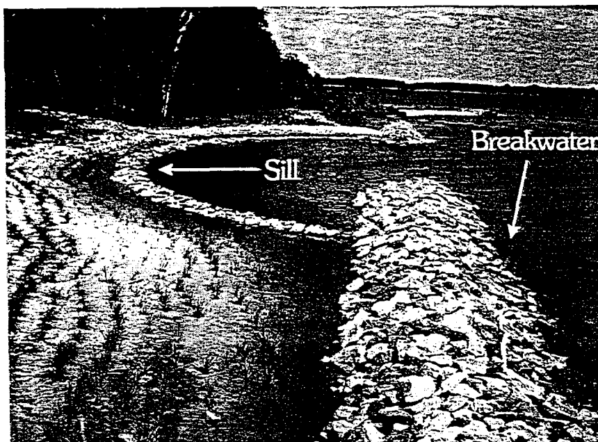
Stone sill with connecting breakwaters, sand fill, and marsh implantation on the Choptank River, Talbot County, Maryland shortly after construction
