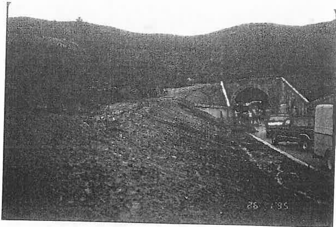
Figure 1. West portal of Baker-Barry Tunnel showing berm and tunnel top subsites following repair and recontouring of soil. Photo taken in 1995 prior to revegetation. Photo by L. Nelson.
