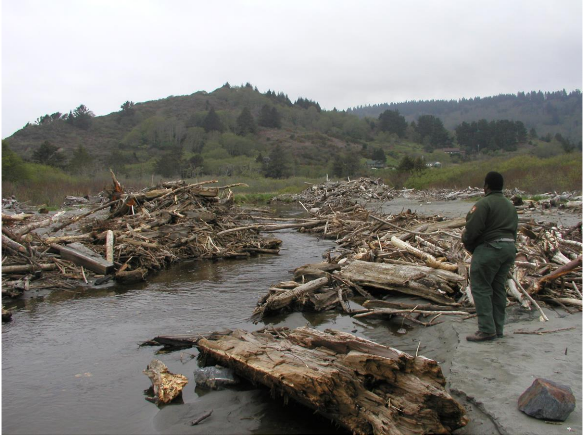
Figure 9. North Slough outlet channel on March 31, 2003 after clearance of the channel of woody debris by adjacent landowner (looking north). Wood was moved to the banks of the channel to allow water to flow unimpeded. (RNSP)
